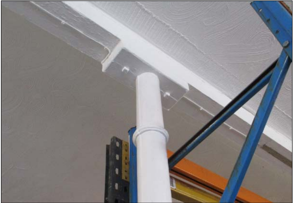
11. One of the remaining steel columns
