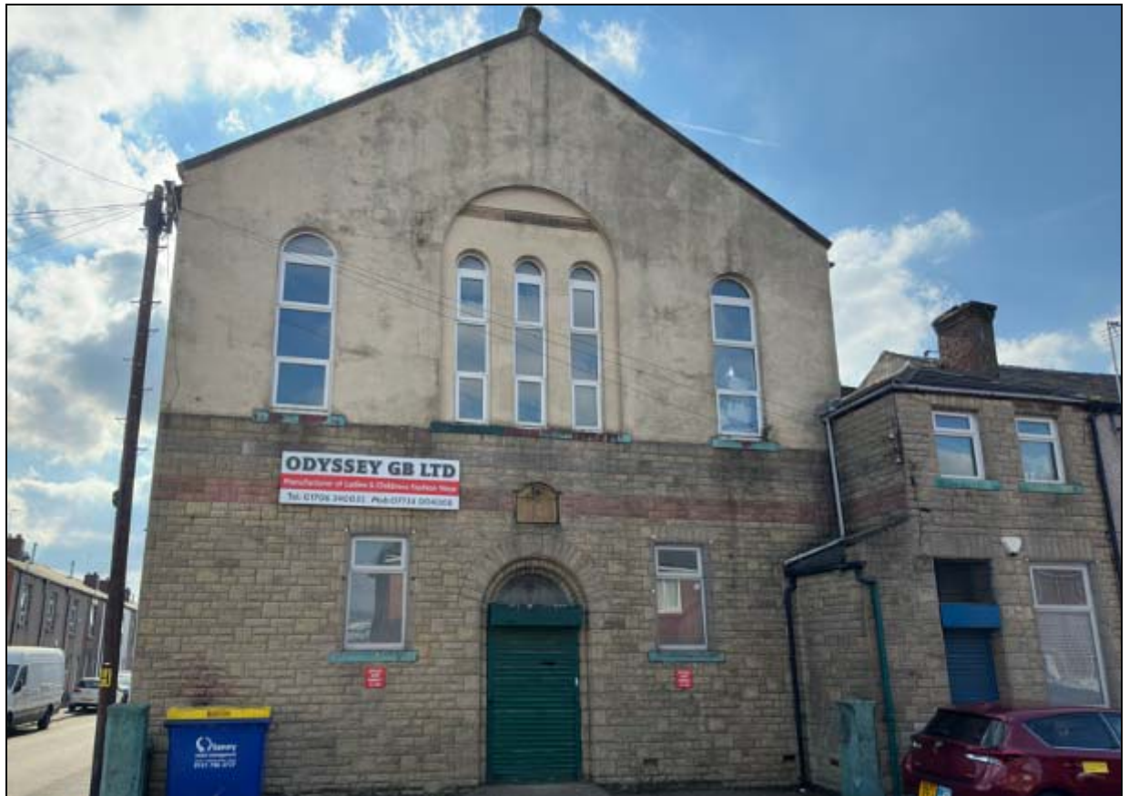
4. The original school building of 1875 and early 20 th century two-storey extension on right
