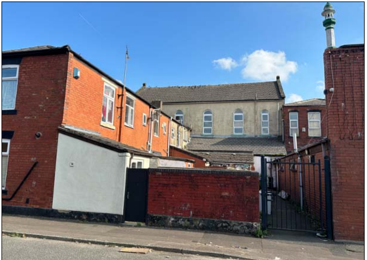
2: The building viewed from the west, beyond terraced properties on Durham Street
