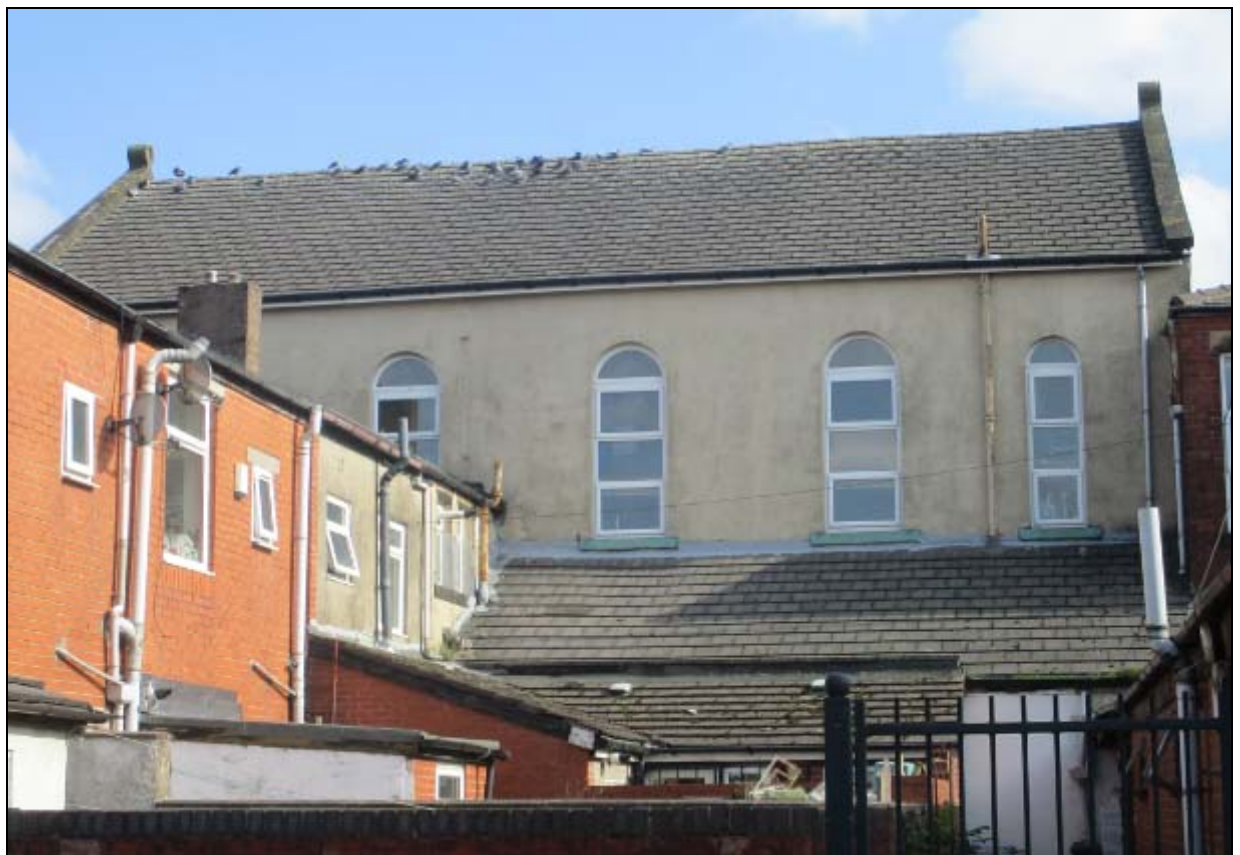
7. West side elevation, viewed from Derby Street
