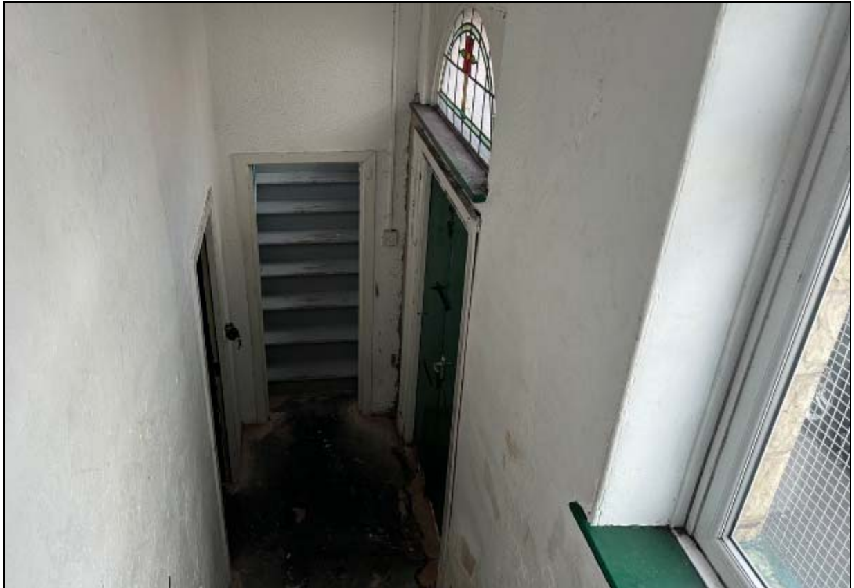
12. Entrance lobby and staircase
