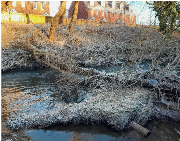
Photograph 5: Section 1 fallen tree in the channel
