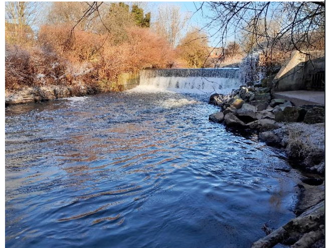
Photograph 10: Section 2 upstream view of weir and outfall
