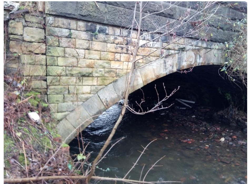
Figure 14 Bridge as viewed from the Site.
