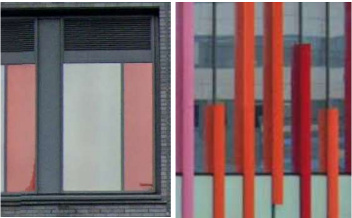
Existing orange transparent film Existing coloured fins
