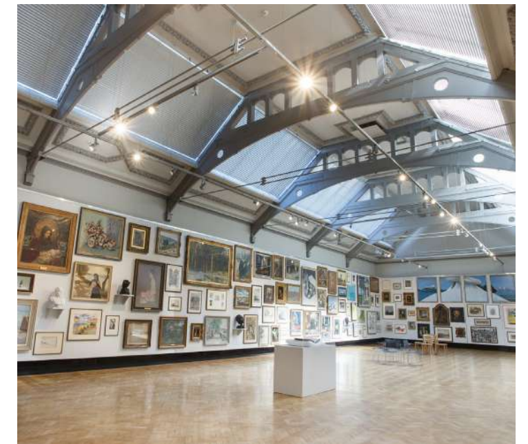
Trusses, main gallery space
