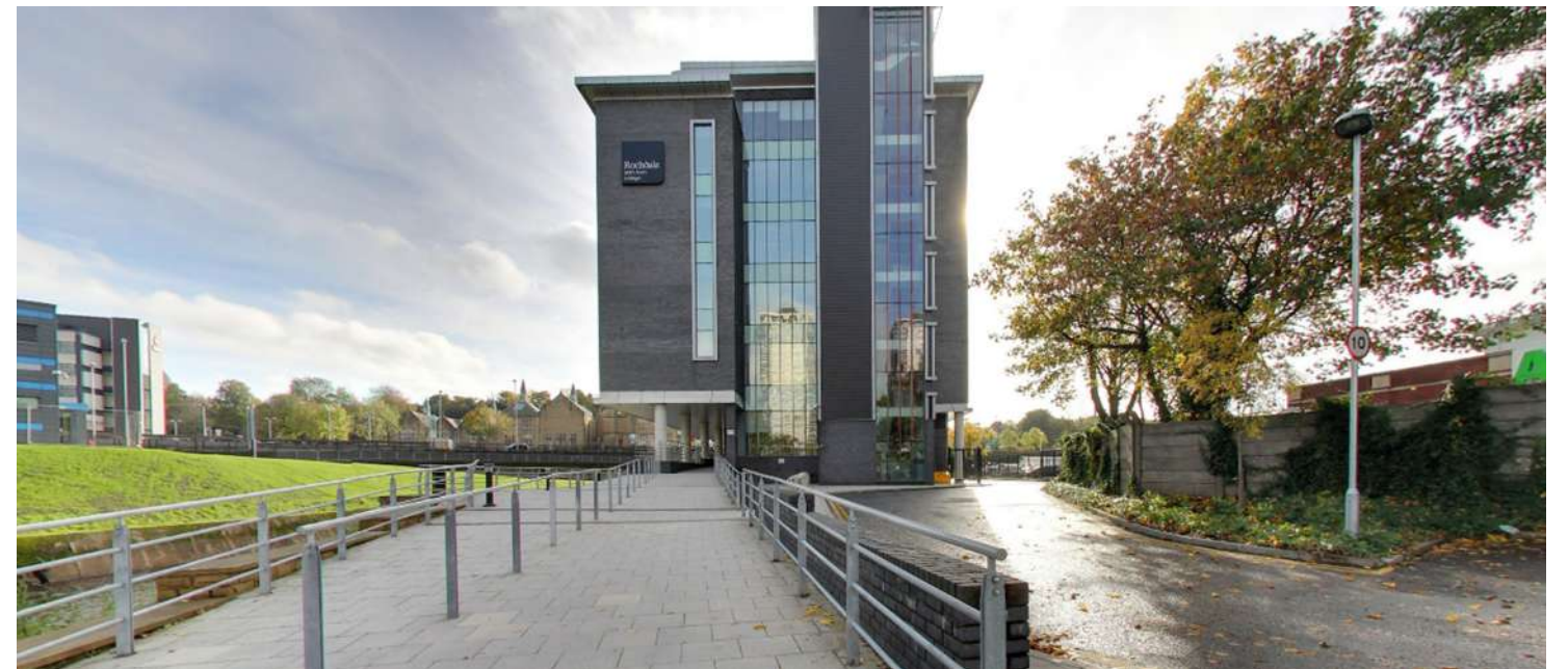
Approach from the North to the existing Rochdale Sixth Form College entrance, Source: Google Maps
