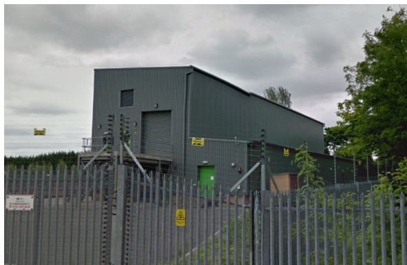
Equipment enclosure - Rochdale Power Station - metal cladding
