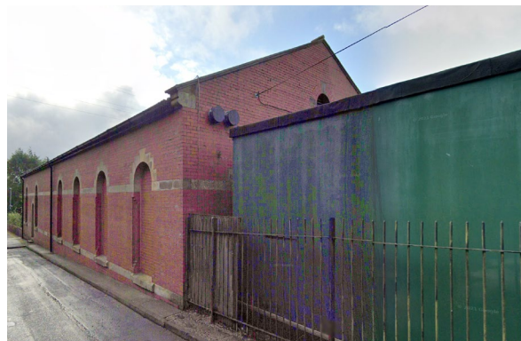
Commercial property - Clay Lane - red brick with sandstone
