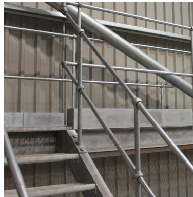
Galvanised tubular handrails and galvanised decking with steps
