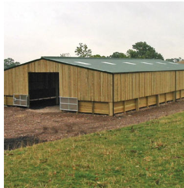
Natural timber close-boarded cladding to barn structures
