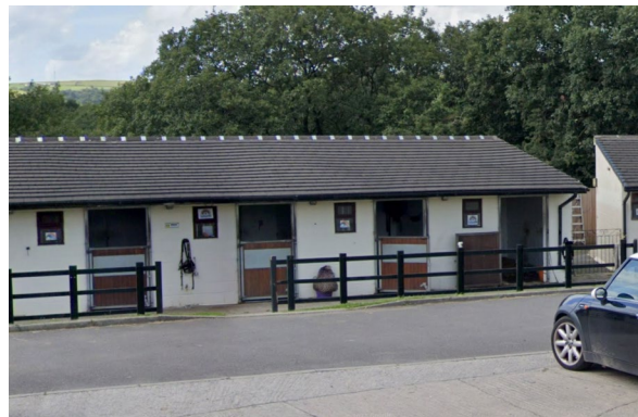
Waterloo Farm - stables - render with concrete tile roofing
