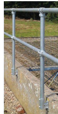
Galvanised tubular handrails and galvanised decking with steps
