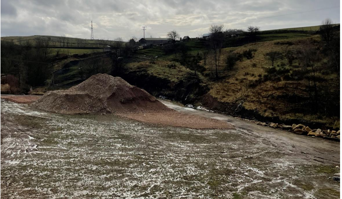
Demolition crush which has now been removed from Site.
