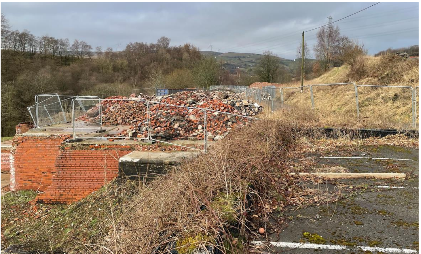
Demolition materials separated for removal.
