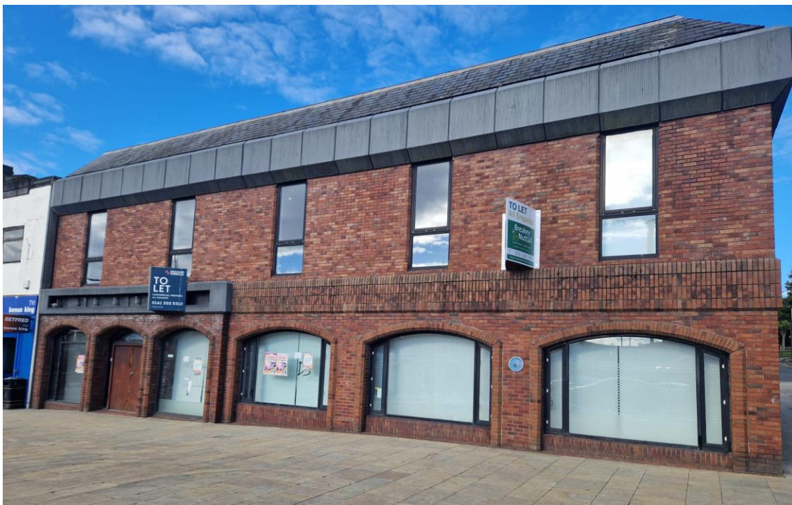
Fig. 2: East Elevation of the Building facing Long Street.
