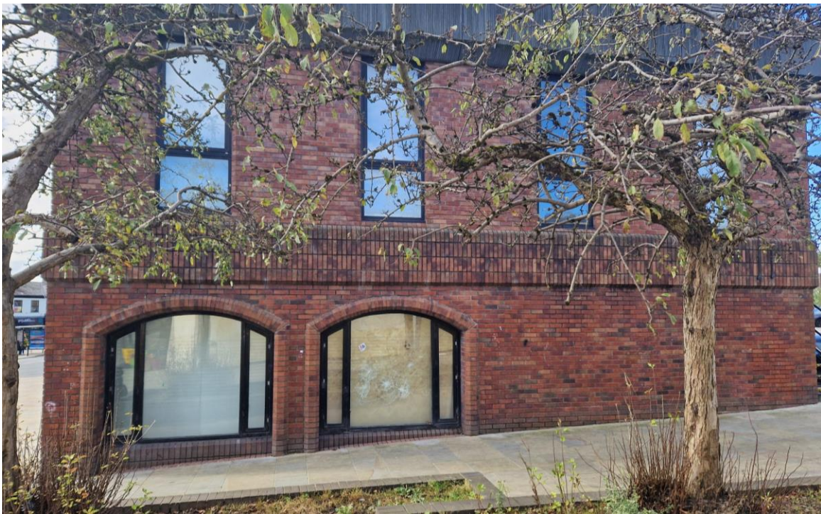
Fig. 4: North Elevation of the building.
