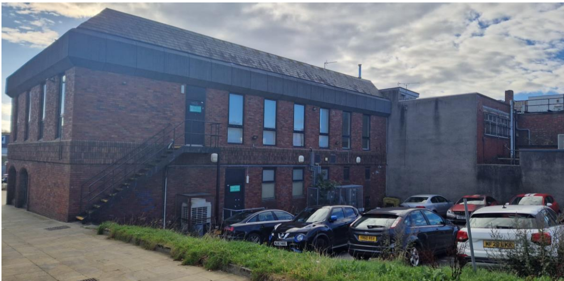
Fig. 3: West Elevation of the building and adjacent Car Park.
