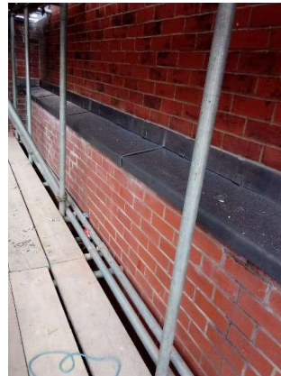
Reading room offset detail flashed
