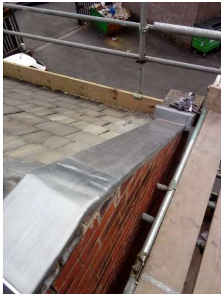
Coping dpc installed ready for coating with bitumen and sand
