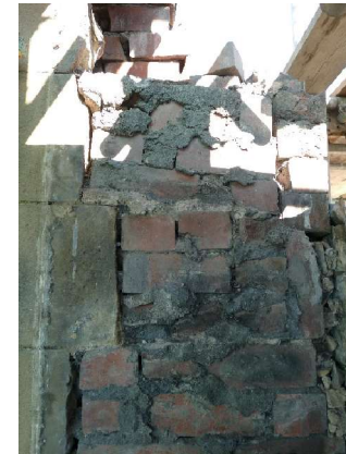
Condition of gable brickwork assessed
