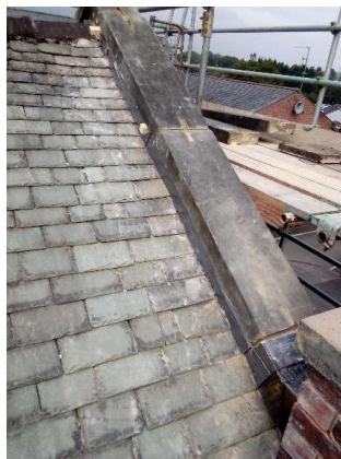
Coping re-installed above meeting room
