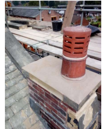
Chimney repaired and re-constructed
