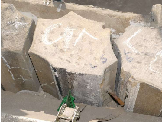
Assessment of stone repairs
