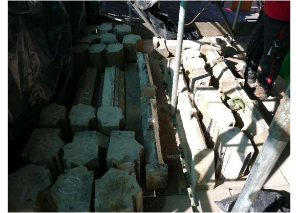
Stonework fully inspected and laid out for re-installation
