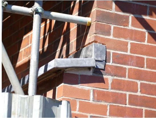
Renewed and improved flashing detail to the offset to the reading room wall.
