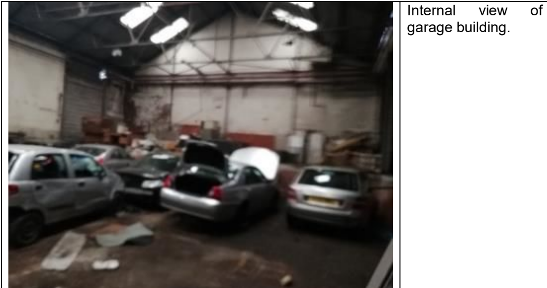
Plate 2-7: Site Reconnaissance: Tack Lea Works.
