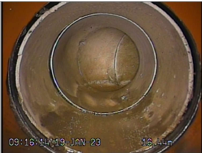
Open joint large
