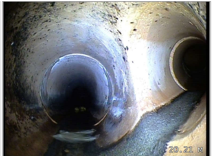
Junction at 3 o'clock, diameter 100mm
