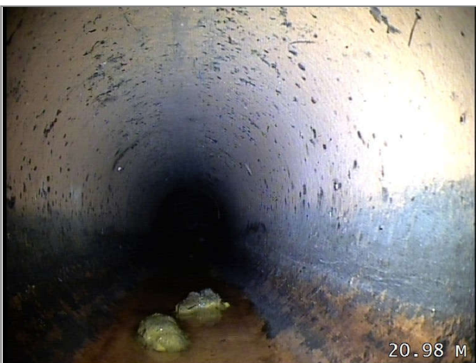
Other settled deposits 5% cross-sectional area loss - Remark: FOUL WASTE DEPOSITS
