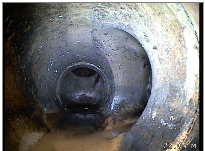
Junction at 3 o'clock, diameter 100mm
