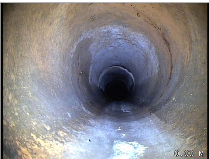
Start node type, manhole, reference MH 08
