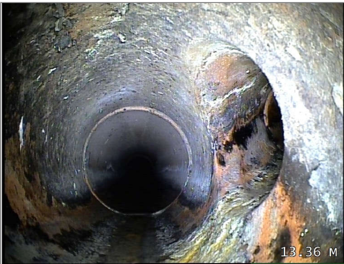
Junction at 3 o'clock, diameter 100mm
