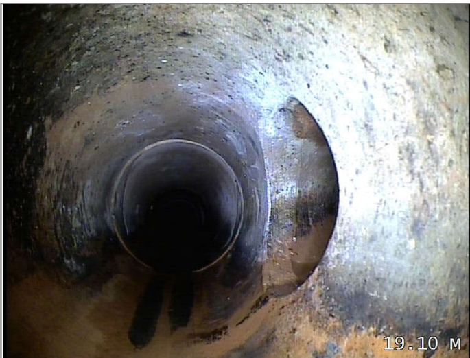
Junction at 3 o'clock, diameter 100mm
