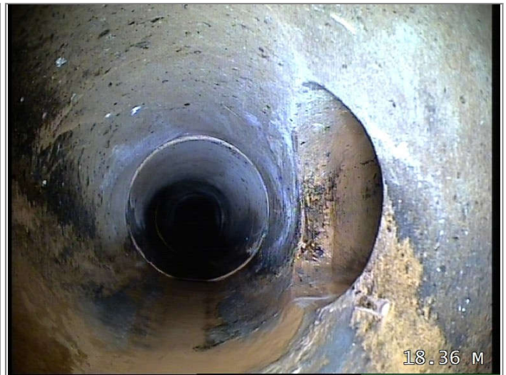
Junction at 3 o'clock, diameter 100mm
