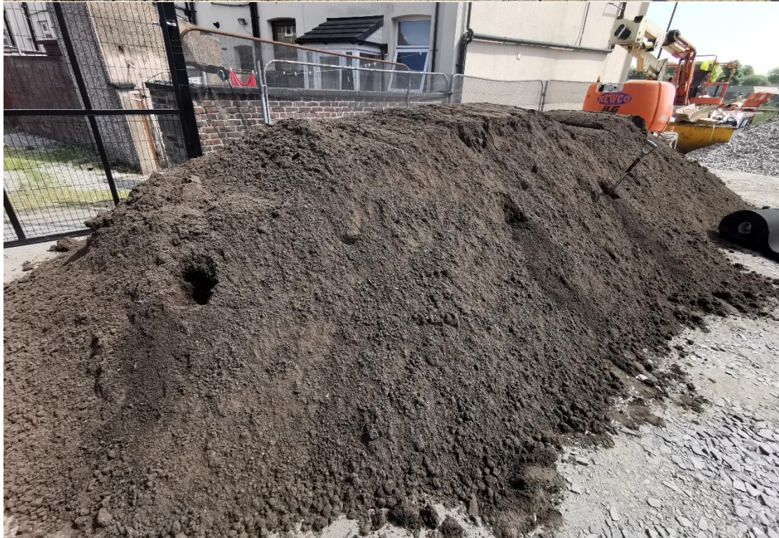
Topsoil import stockpile, virgin quarried sand & MOT in the b/g
