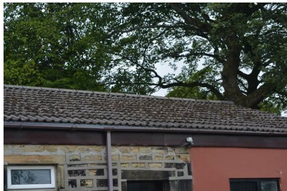
Figs. 5 & 6 Gaps beneath ridge tiles (stables)
