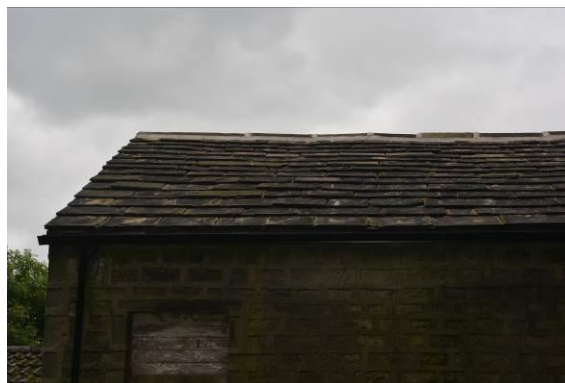
Figs. 3 & 4 Raised tiles on barn roof
