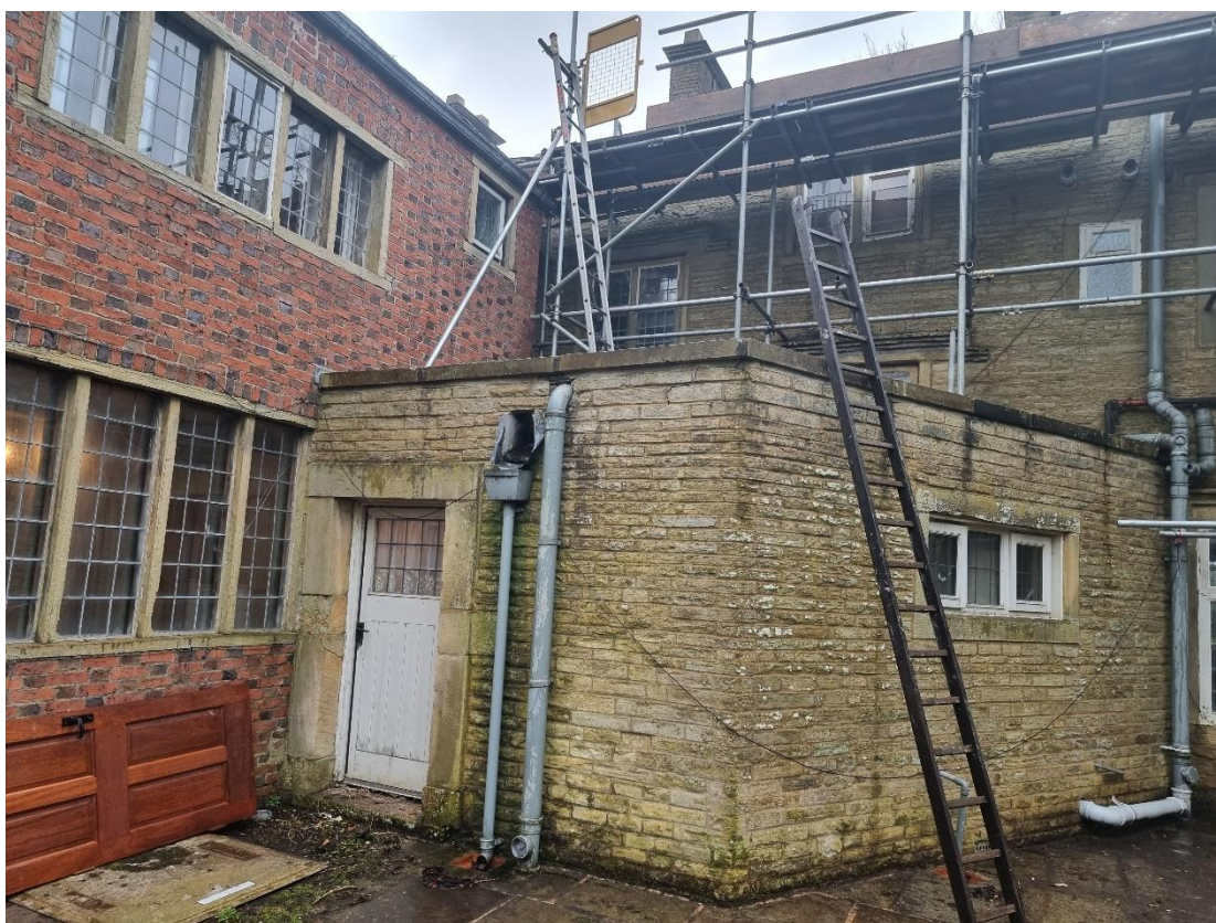
Fig.13: The single storey addition adjoining the ring wing and main range of the house dates to between 1890 and 1908, based upon historic map regression of the plan form. This also makes it likely that it was built in the same phase the southwest corner of the house, seen below.
