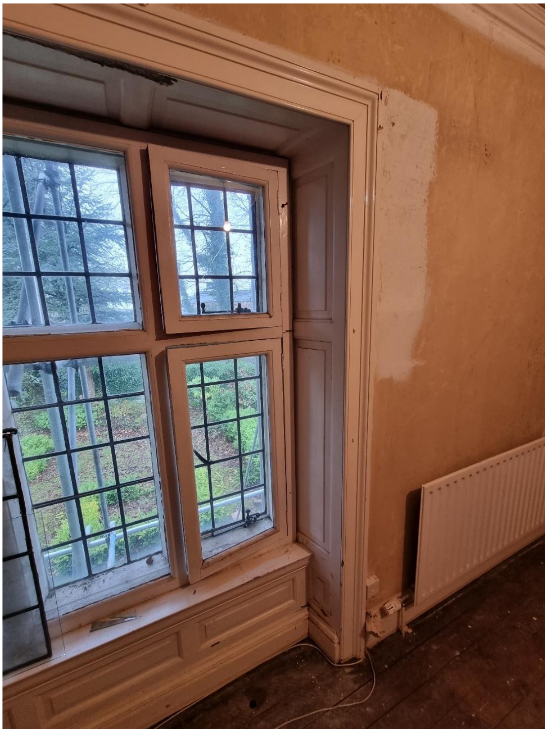
Fig.32: Typical example of secondary glazing used in multiple places throughout the property.
