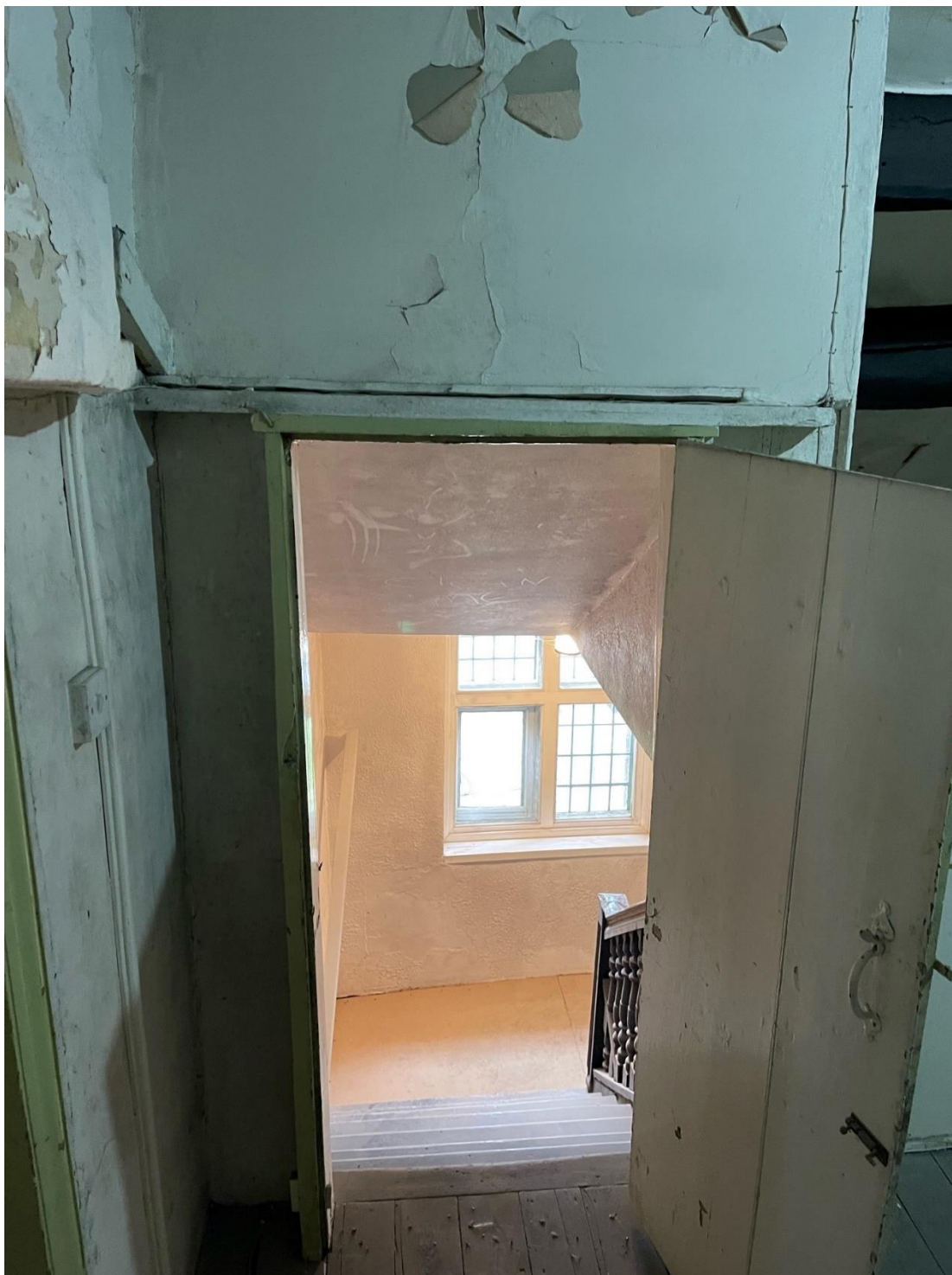
Fig.28: View looking down from the attic door to the half-landing, window, and modern plasterboard bulkhead.
