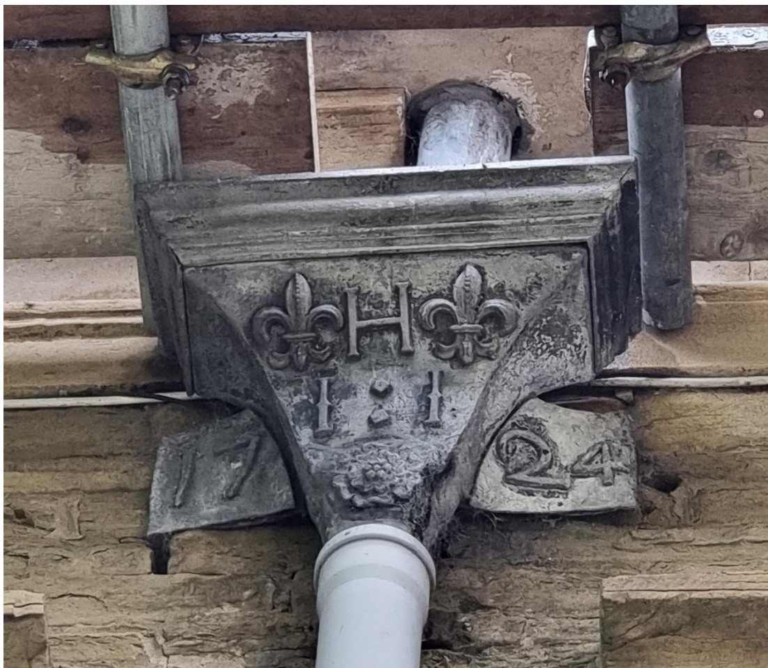
Fig.16: The rainwater hopper stamped with the date 1724.
