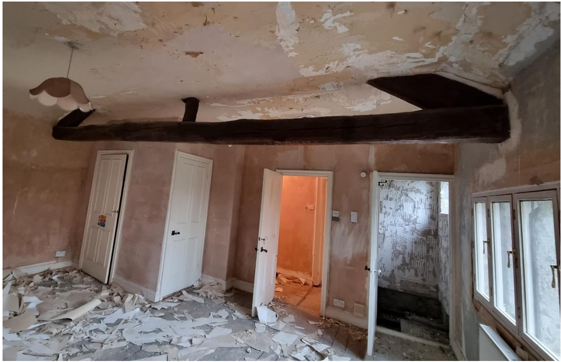
Fig.25: Image shows an exposed tie beam and principal rafters forming a truss and is located in Bedroom 6 (see plans) which forms part of the rear projection. The tie beam would suggest the ceiling was a post construction addition.
