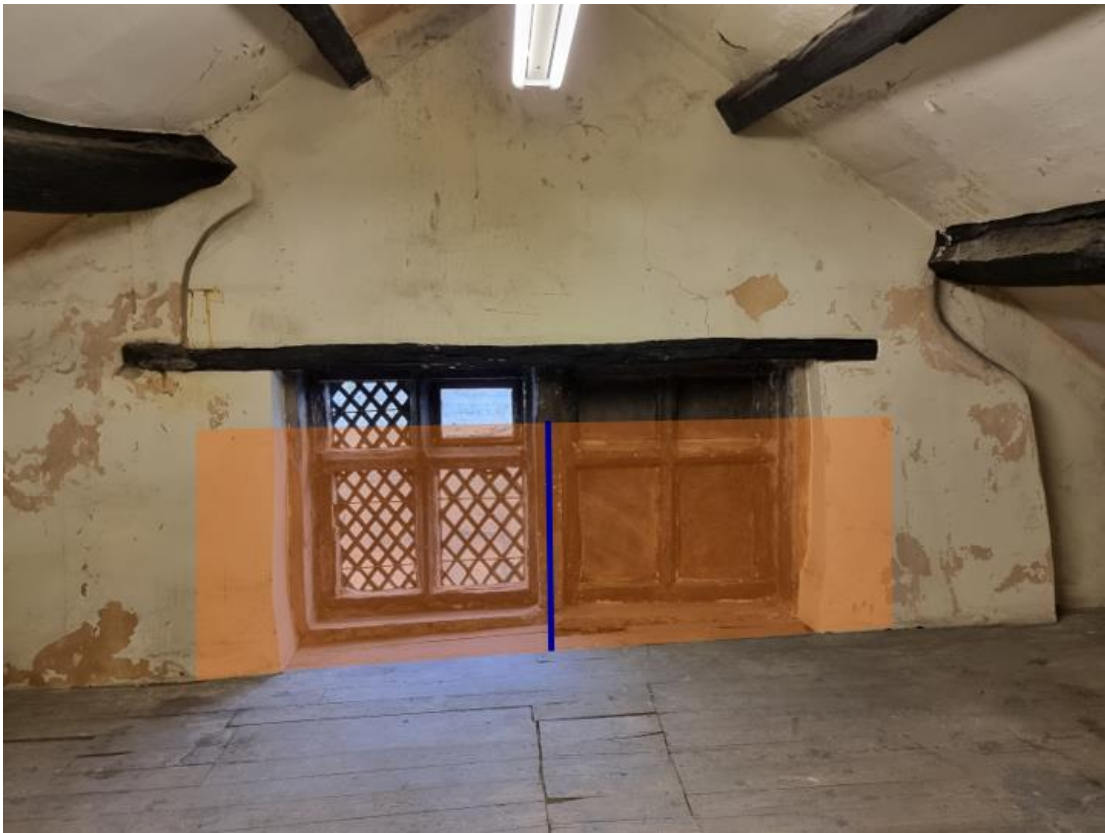
Fig.38: The diamond leaded window (and blocked up counterpart) - the orange overlay denotes the protective glazed screen to be installed for health and safety reasons.
