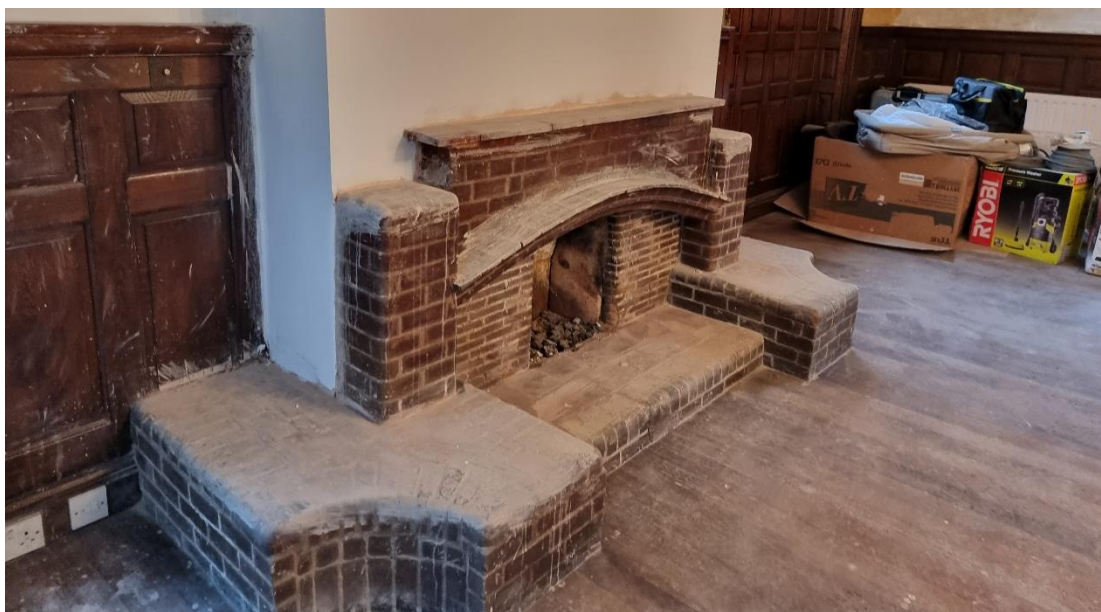
Fig.24: An Arts and Crafts style fireplace c.1900 in the addition built in the same period.
