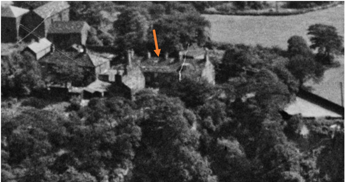
Fig.8: Aerial photo, taken 1934. The rear (north elevation) of Old Falinge is seen in the centre of the photo.
