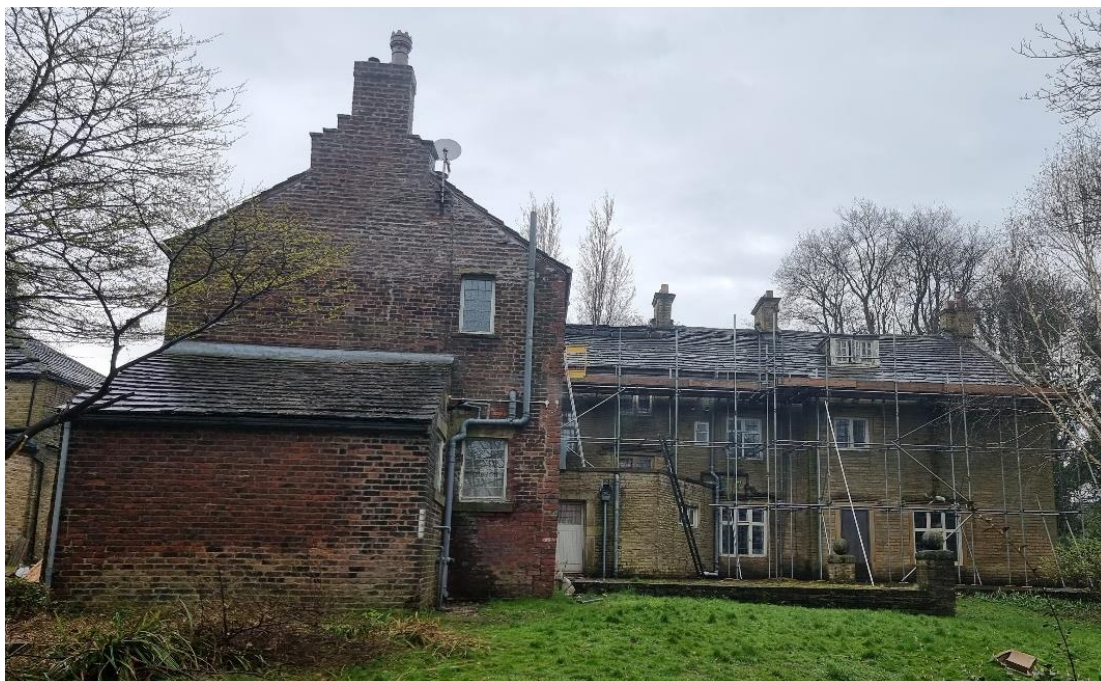
Fig.12: The rear (north) elevation of Old Falinge.
