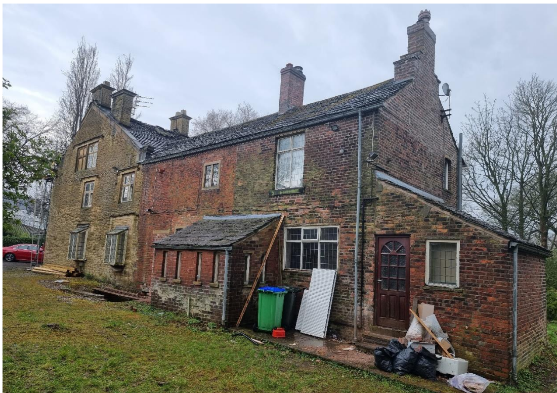
Fig.10: The east elevation of Old Falinge, April 2022. This elevation exhibits a wide variety of brick types and bonds owing to the periods of construction and reconstruction.
