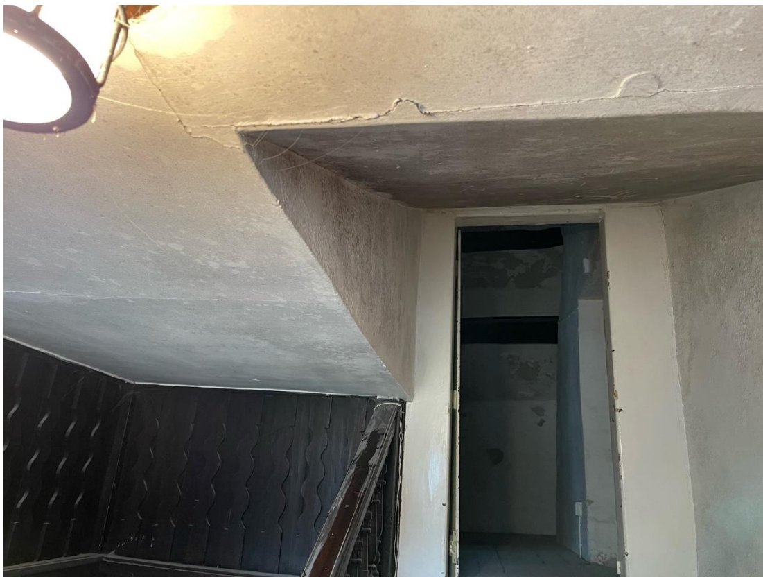
Fig.27: The bulkhead viewed from within the stairwell, looking up into the attic.
