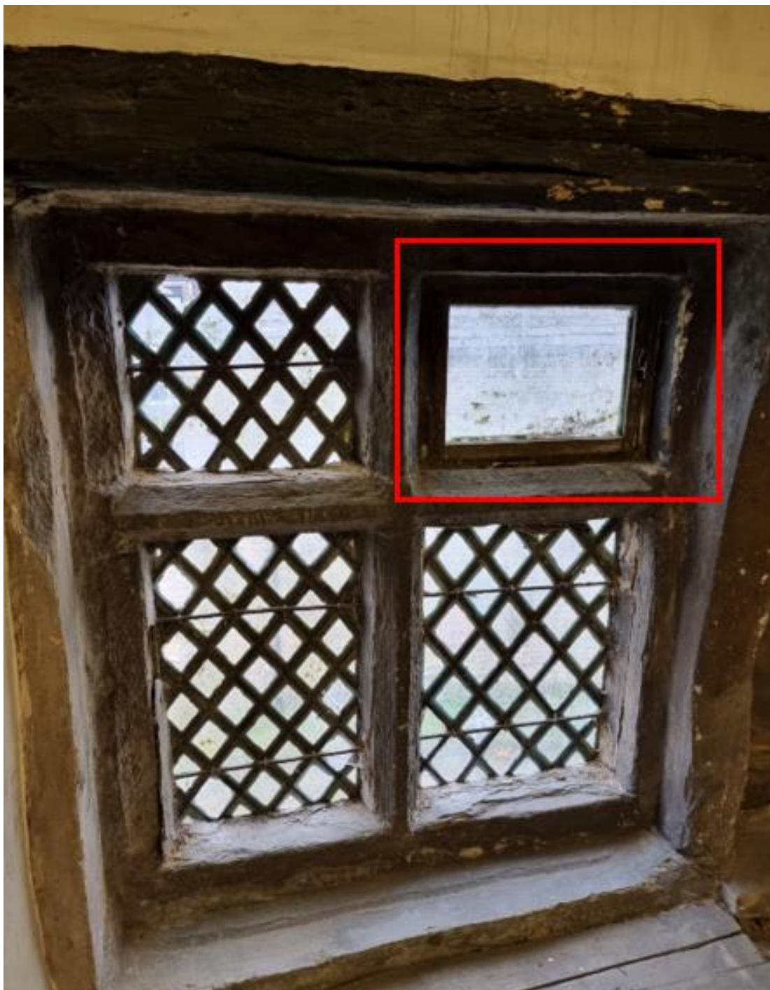
Fig.39: The diamond leaded window features a modern casement unit to the top corner which is to be replaced with a leaded pane to match the rest of the window.
