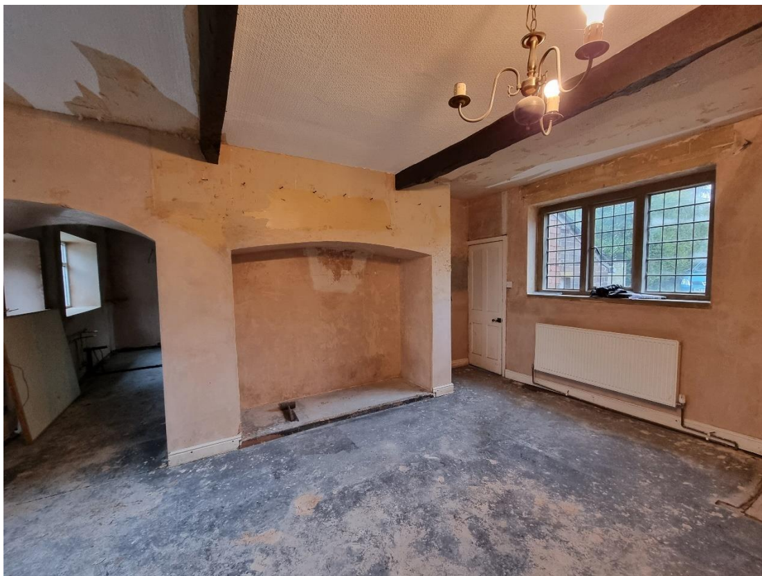
Fig.22: Looking through from the breakfast room to the kitchen beyond on the ground floor of the brick rear wing.
