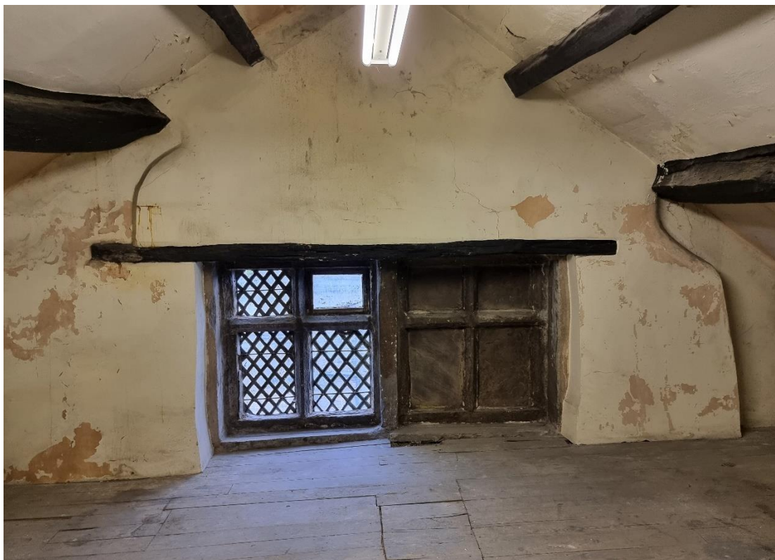
Fig.18: An identical window to the right was blocked in with stone, probably also in the 18 th century in response to the window tax in force at the time. This corner of the building is the oldest part of the house, and the historic beams can also be seen in this image.
