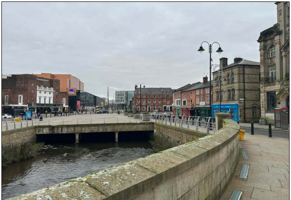
2. More distant view from the west, by the culverted River Roch
