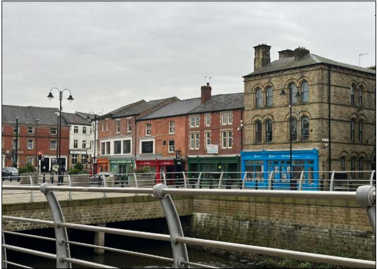
7. The property viewed across the River Roch. Its contribution to the conservation area stems primarily from its group value with the rest of the South Parade row
