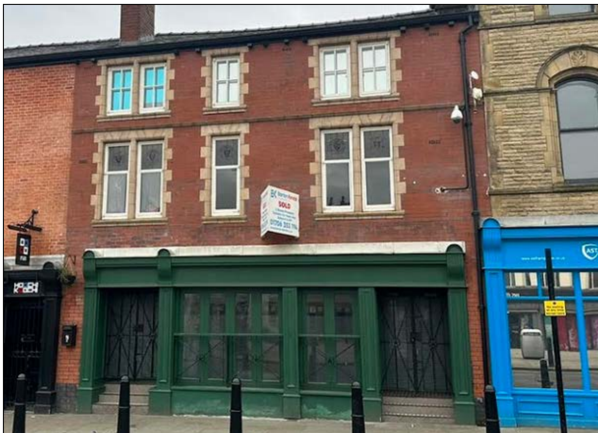
4. Present appearance of the front elevation
