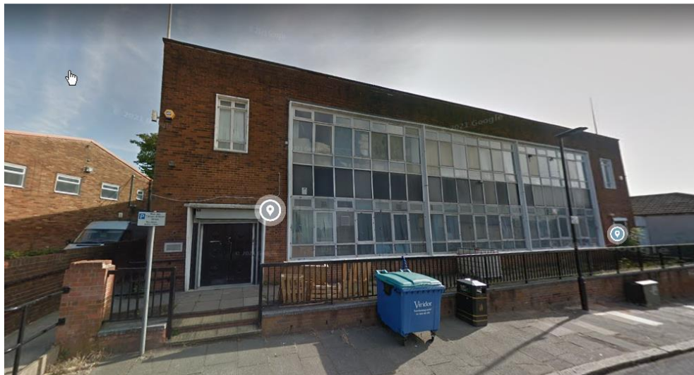
Figure 1 Street view of site
