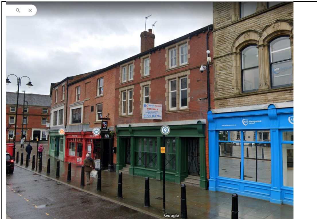
View of building
