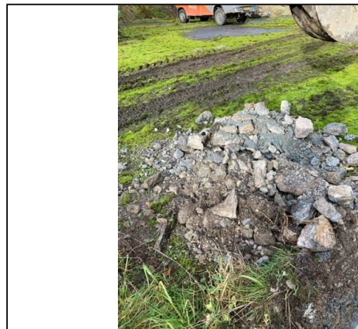
Trial Pit 111 Spoil
