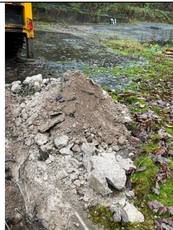
Trial Pit 121 Spoil
