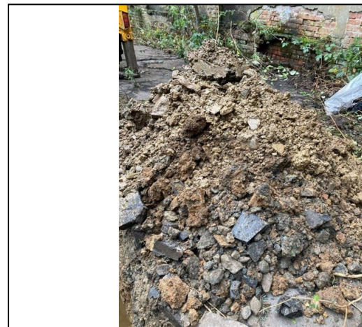
Trial Pit 119 Spoil
