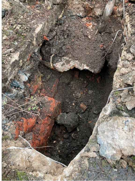
PLATE 4 TP116 EXCAVATION WITH OBSTRUCTIONS
