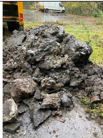
Trial Pit 124 Spoil
