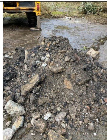
Trial Pit 113 Spoil
