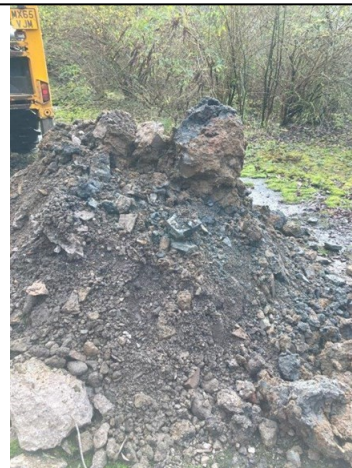
Trial Pit 110 Spoil
