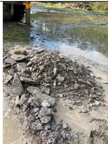
Trial Pit 112 Spoil
