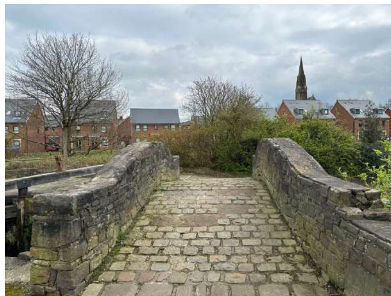
Figure 4.2: Rochdale Canal Towpath Bridge (April 2024)
