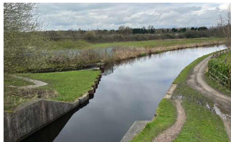
Figures 3.2 & 3.3: Views of the Application Site (April 2024)
