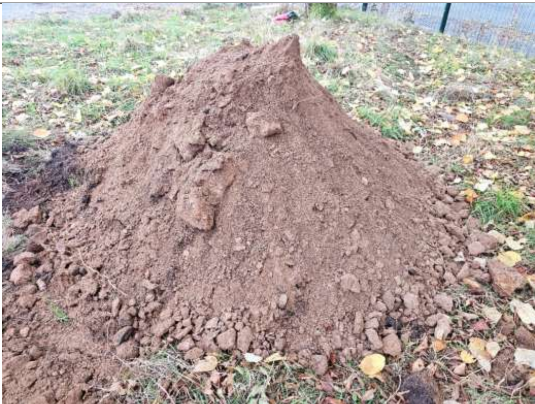
Trial Pit S1 – excavated spoil
