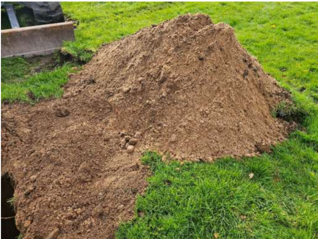
Trial Pit S5 – excavated spoil
