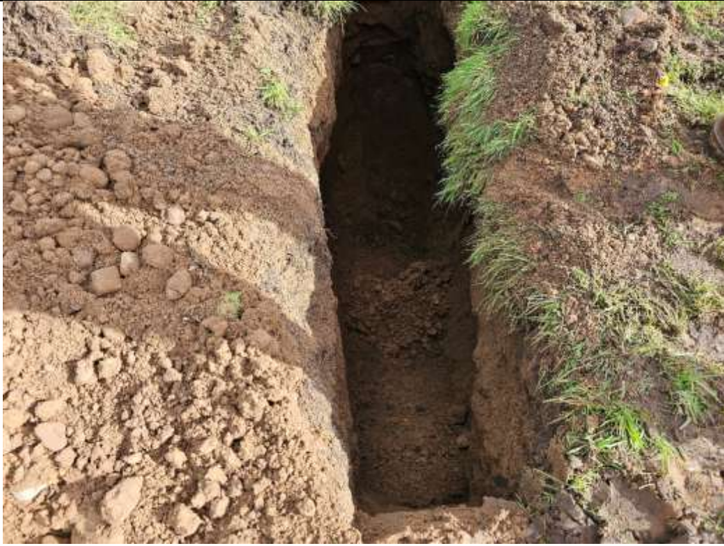
Trial Pit S3 – after excavations
