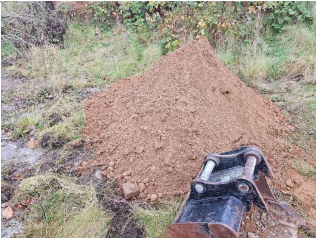
Trial Pit S2 – excavated spoil
