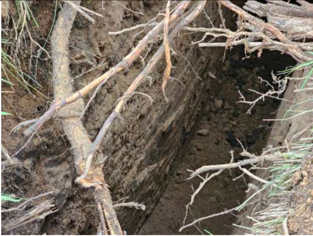
Trial Pit S1 – after excavations
