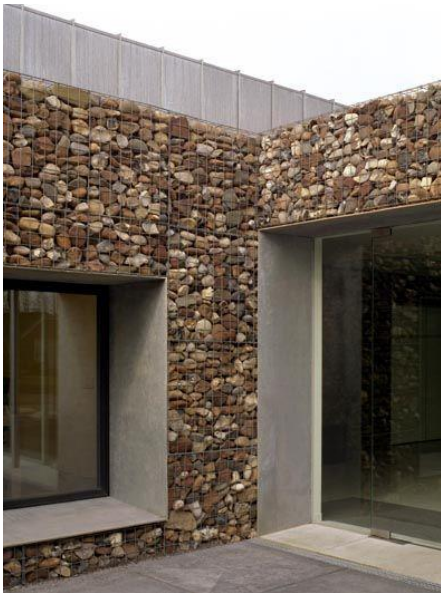
deep reveals to super-insulated walls
