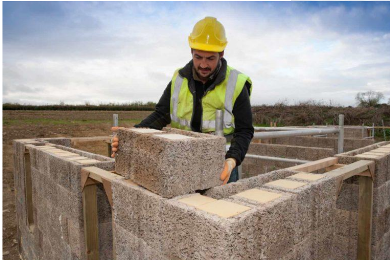
Durisol woodcrete blocks (made from recycled wood)
