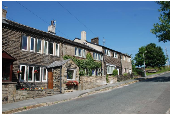
cottages to the east of the site
