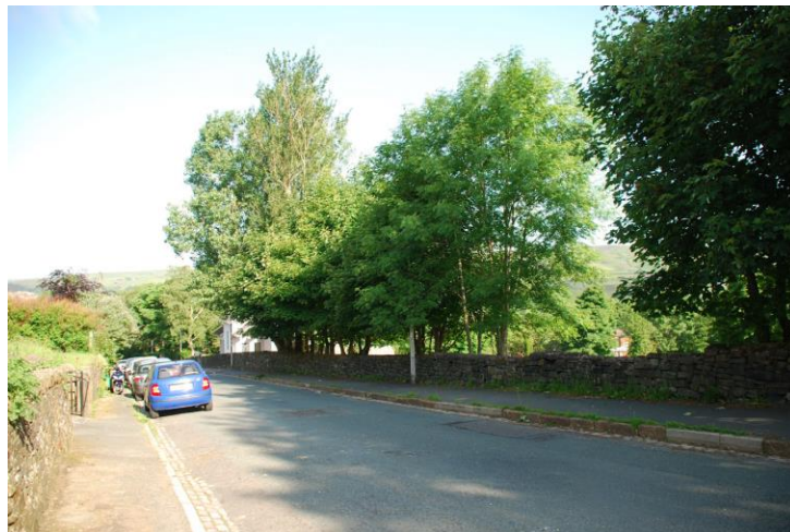
natural stone wall to site boundary
