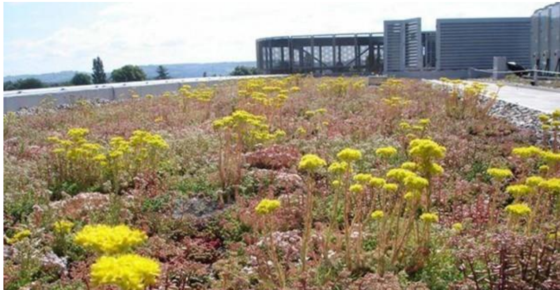
sedum roof with high level of insulation in the build up
