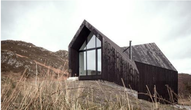
charred timber cladding
