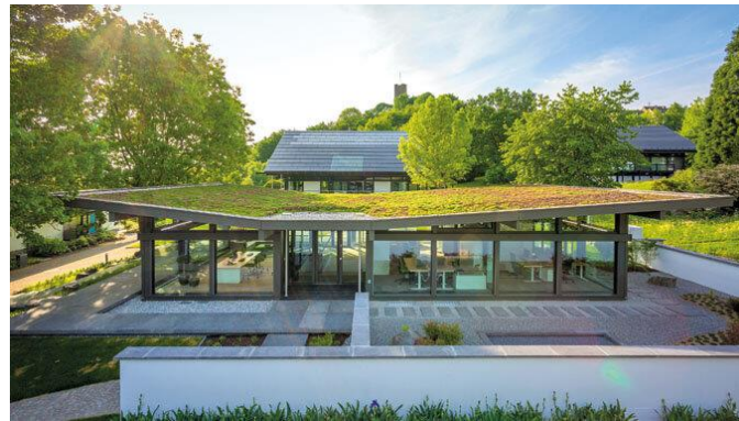
Sedum roof with metal fascia (zinc)
