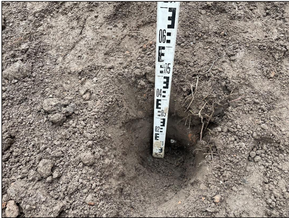
View of Plot 6 rear garden exposing geotextile membrane at base of excavation. Validated on 13 th March 2024.
