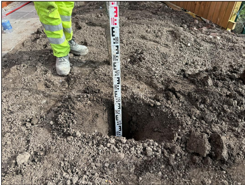
View of Plot 5 side garden excavated to a depth of 0.60m. Validated on 5 th March 2024.
