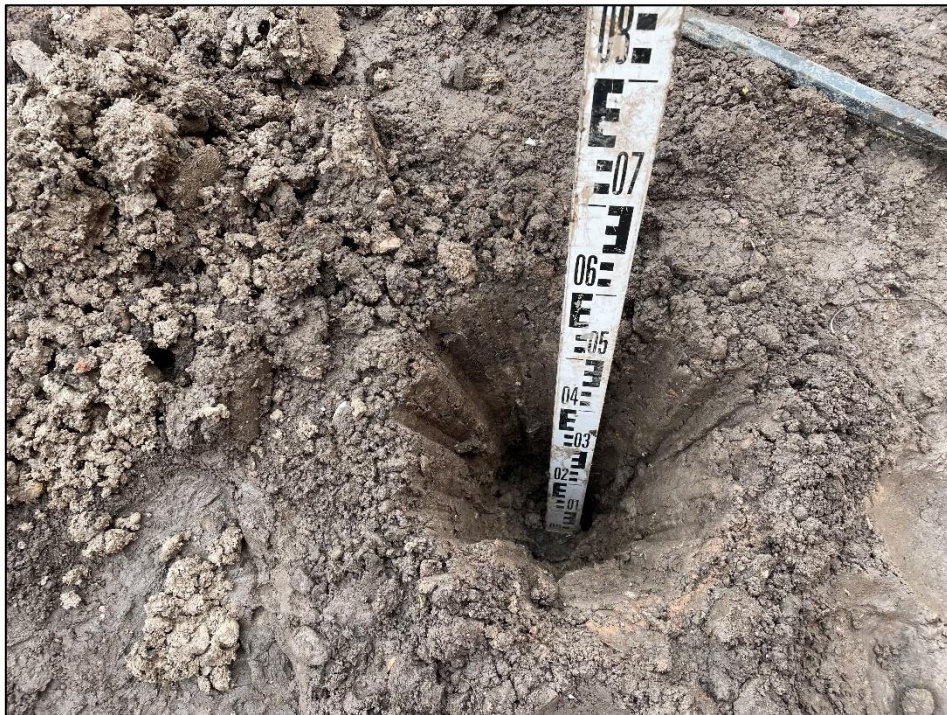
View of Plot 6 side garden excavated to a depth of 0.60m, exposing geotextile membrane at base at 0.60m. Validated on 13 th March 2024
