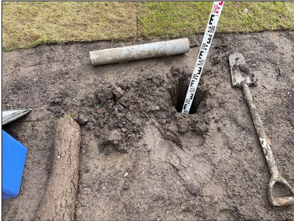
View of Plot 1 front garden excavated to a depth of 0.60m exposing geotextile membrane at base. Validated on 27th March 2024
