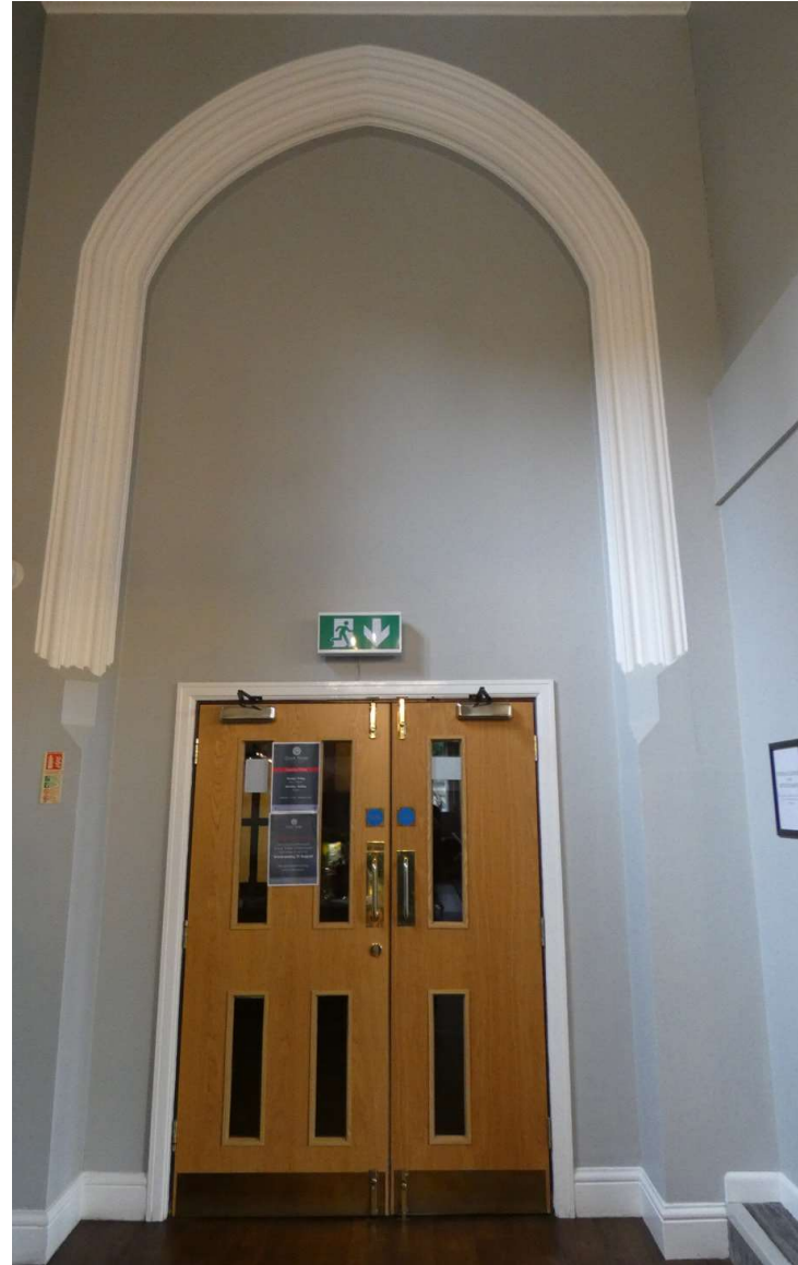
G6. Door in north wall to G2h.
