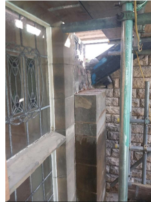
Dismantled entrance gable buttress being re-built and tied in for future stability..
