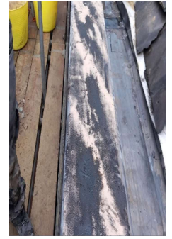
Copings and gutter flashing, facing the Old Police Station, flashed and re-installed. Brickwork raked out ready for re-pointing.
