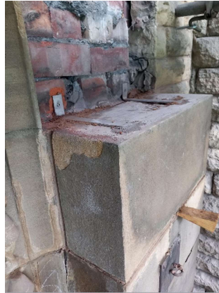
Dismantled entrance gable buttress being re-built and tied in for future stability..
