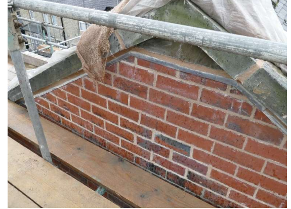
Completed coping, flashing detail and pointing to the meeting room roof.
