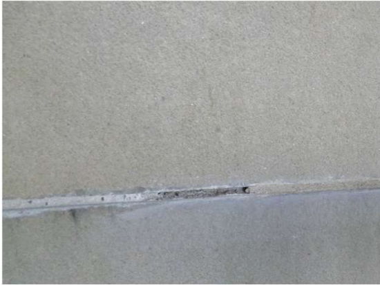
Mortar samples for the stonework. Initial to the left and preferred to the right
