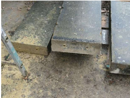
Copings to the flat roof parapet prepared and drilled to receive locating dowels.
