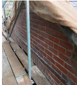
Reading room gable raked out ready for re-pointing.
