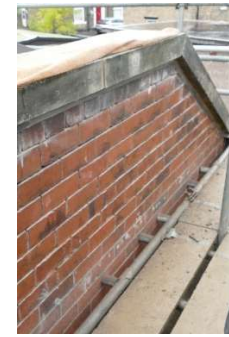
Copings and gutter flashing, facing the Old Police Station, flashed and re-installed. Brickwork raked out ready for re-pointing.
