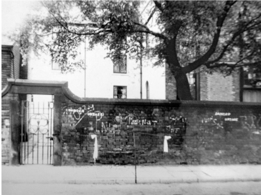
Fig.15: front wall in c.1971 (photograph in chapel, 2019)
