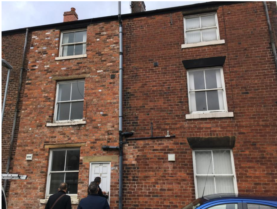
Fig.25: north elevations of No.21 Wilson Street (right) and No.23 (left)
