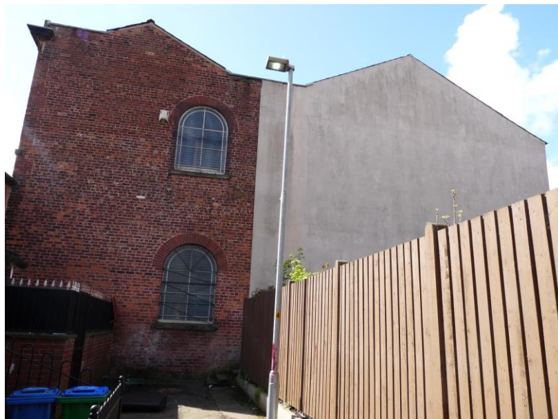
Fig.18: east elevation, with 1848 addition to the left (south)
