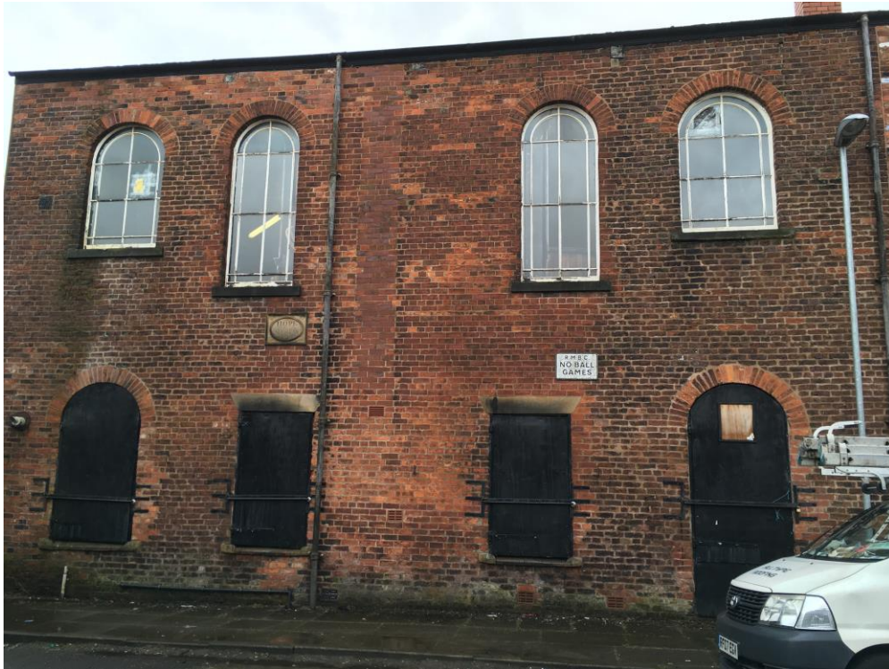
Fig.19: rear elevation from the north
