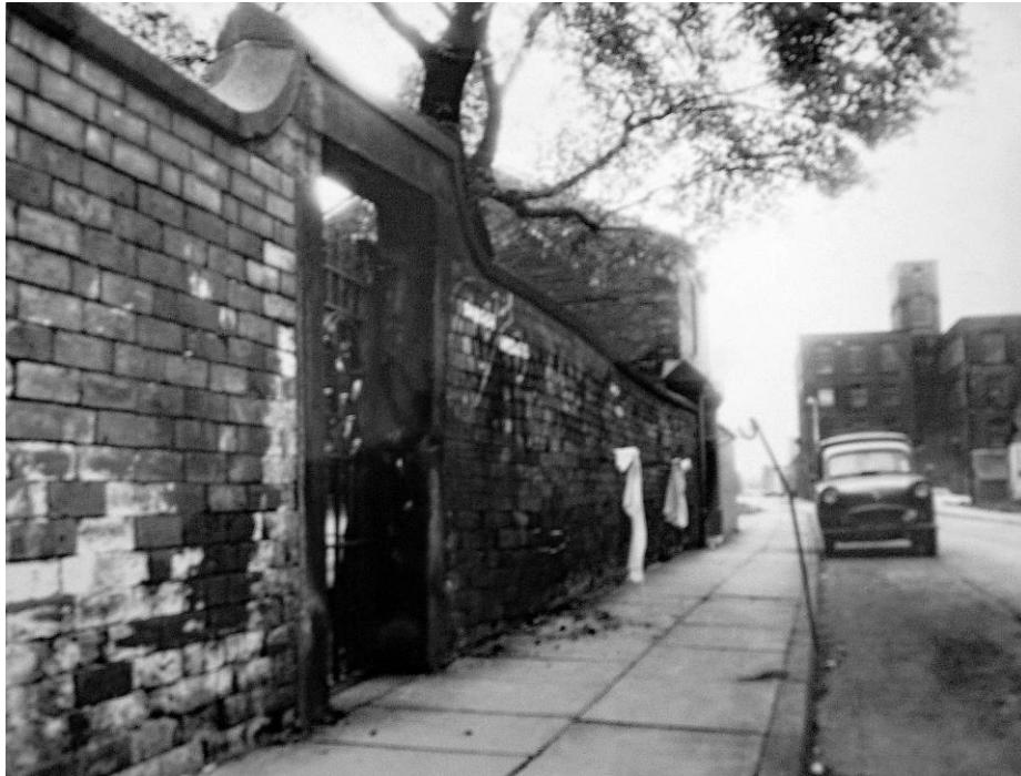
Fig.16: photograph of front wall from the west, c1971 (photograph in chapel 2019)
