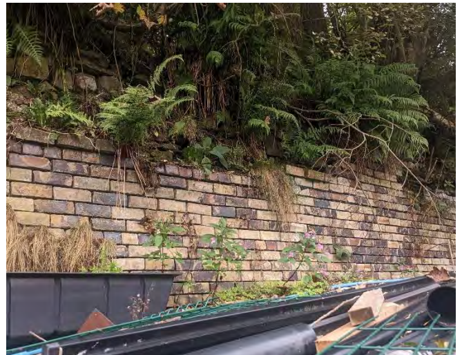
Figure 12 – Retaining walls off-site near the southeastern site boundary, looking east.
