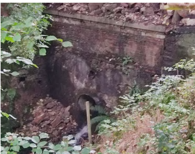
Figure 11 – Looking south, a retaining wall near the northern site boundary, looking south.
