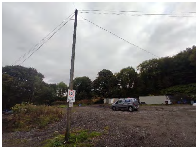
Figure 14 – Overhead power lines noted along the southern and western site boundaries, looking north-east.
