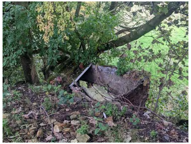
Figure 8 – Historical structures near the northern site boundary, looking north.
