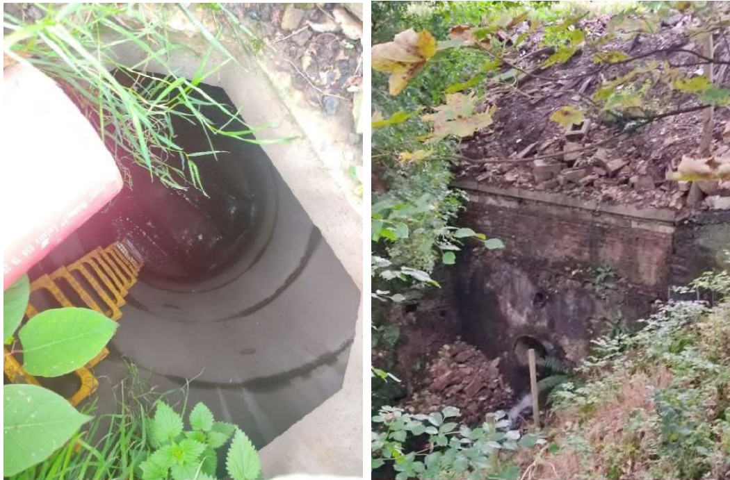
Figure 5: Photographs showing the culvert access point on-site in the western site section (left) and the northern retaining wall where the culvert ends (right).
