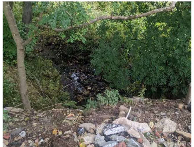
Figure 4 – The exit of the Wicken Hall Clough culvert near the northern site boundary, looking north.
