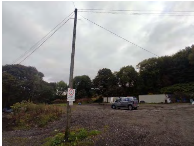
Figure 6: Photograph showing the overhead electricity lines in the southwestern site corner, looking northeast.
