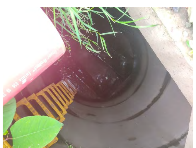
Figure 10 – The on-site culverted stream, at approx. 7.00m depth in the western site section.
