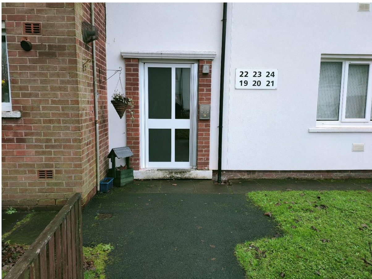
Above – existing access to flats 19-24
