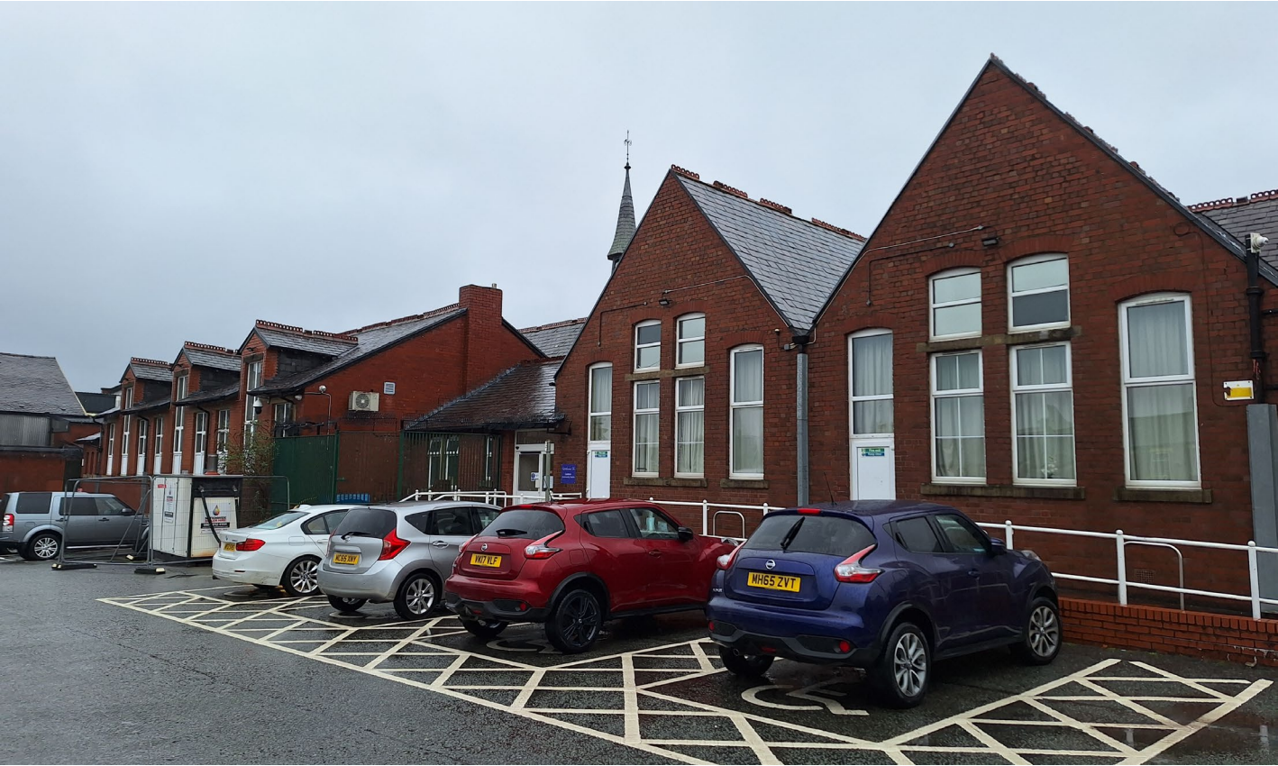
Figure 5. Photograph of Knoll Street elevation taken February 2024 [©Triangle Architects]
