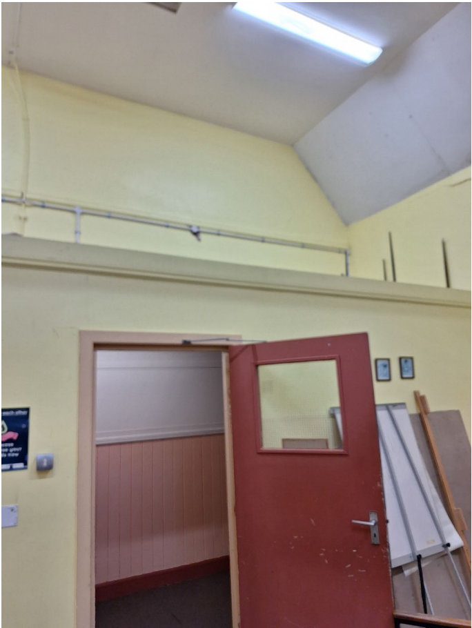
Figures 8 & 9. Internal Photographs showing poor-quality alterations, including additional internal corridor, low grade fire doors, grid ceiling, and evidence of water penetration. [©Triangle Architects]
