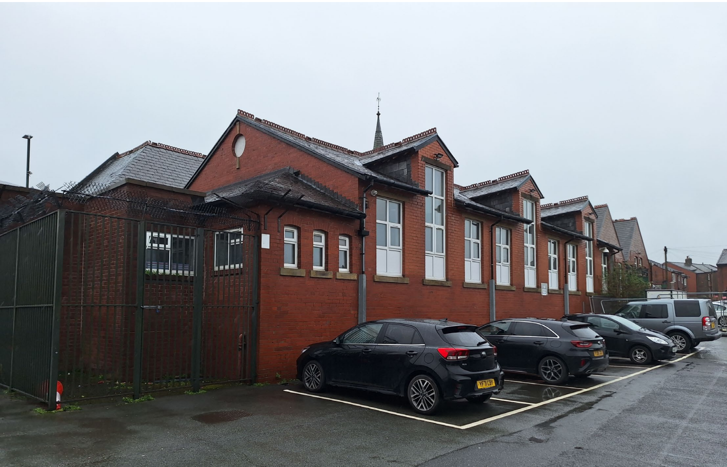
Figure 6. Photograph of Knoll Street elevation taken February 2024 [©Triangle Architects]
