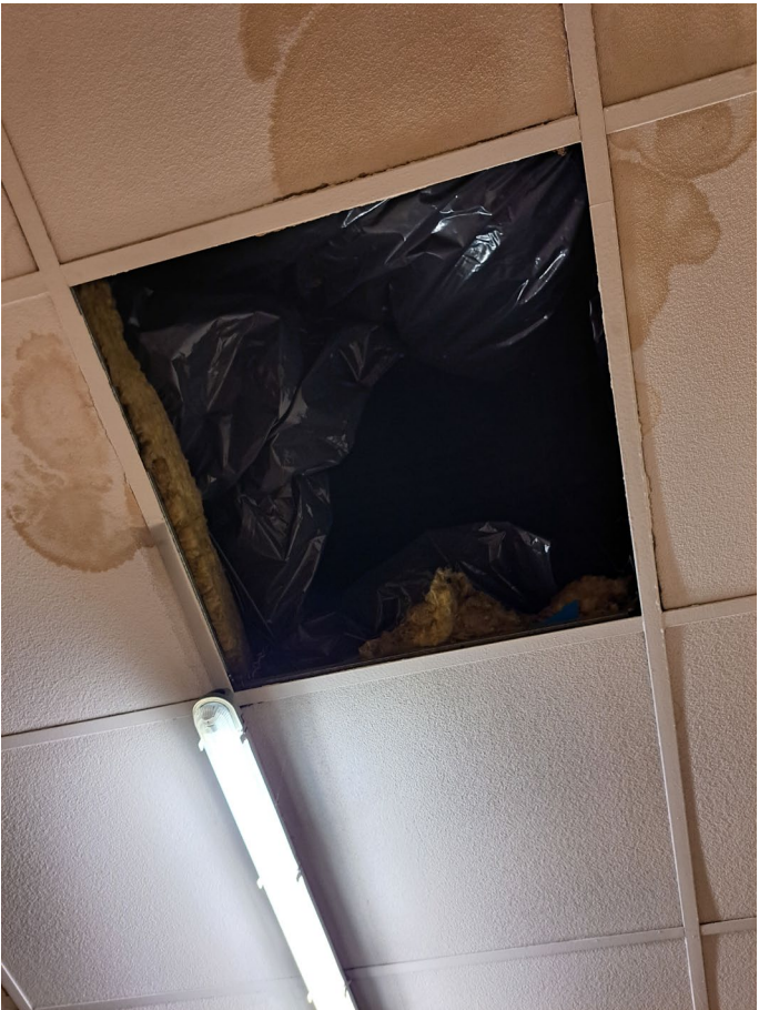
Figures 8 & 9. Internal Photographs showing poor-quality alterations, including additional internal corridor, low grade fire doors, grid ceiling, and evidence of water penetration. [©Triangle Architects]
