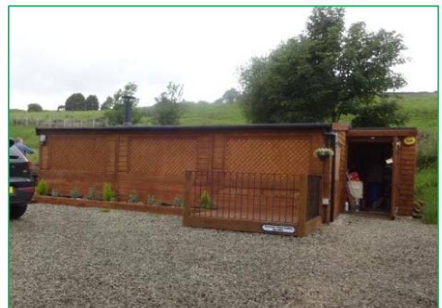
The cabin; developed land sealed surface
