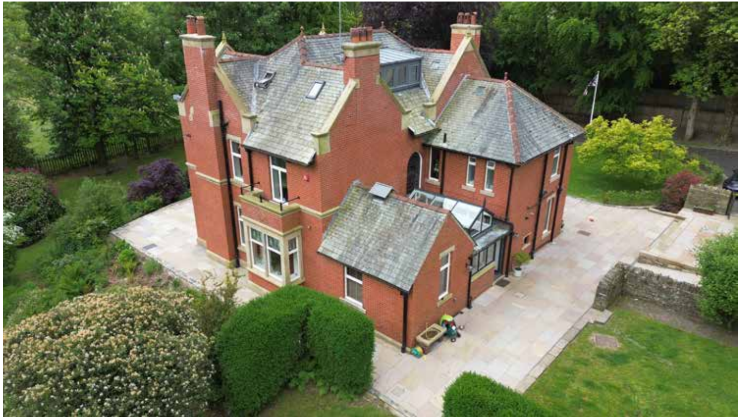
Drone View from north-east corner of site looking south-west
