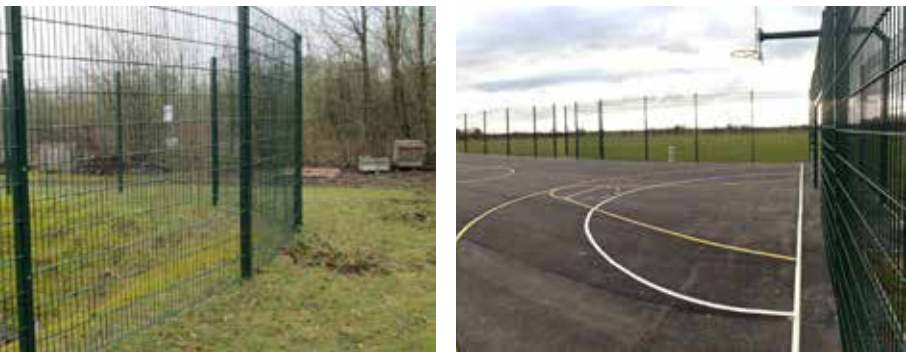
Secure mesh and MUGA fencing (RAL 6005 Moss Green finish) as proposed
