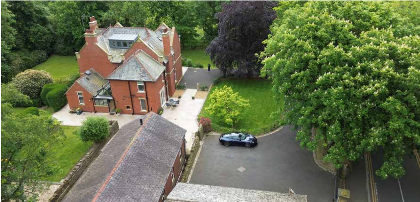
Drone View from north-west corner of site looking south
