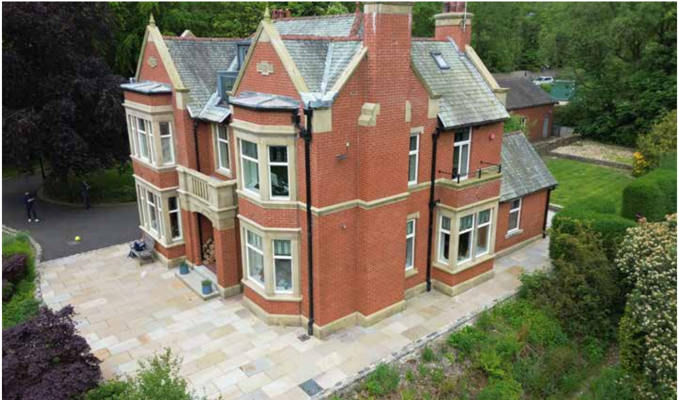
Drone View from south-east corner of site looking north-west
