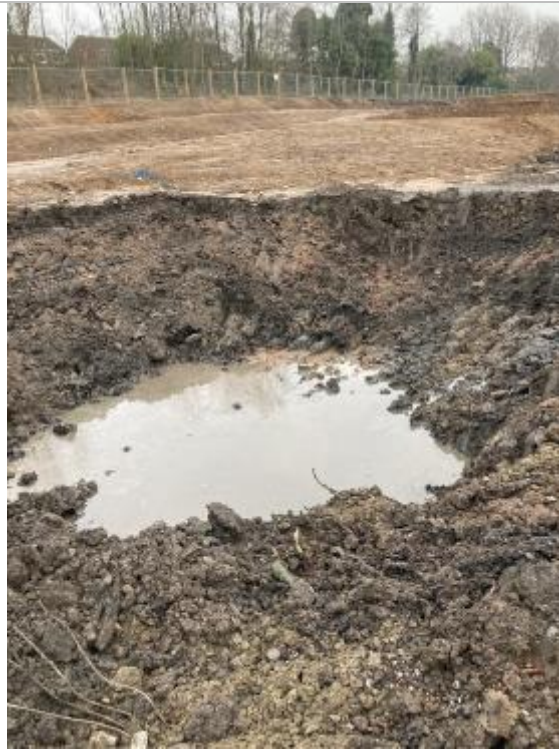
PLATE 37 SUPPLEMENTARY TRIAL PITTING OF IMPACTED SOILS
