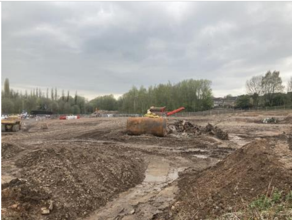
PLATE 40 REMOVAL OF TANK
