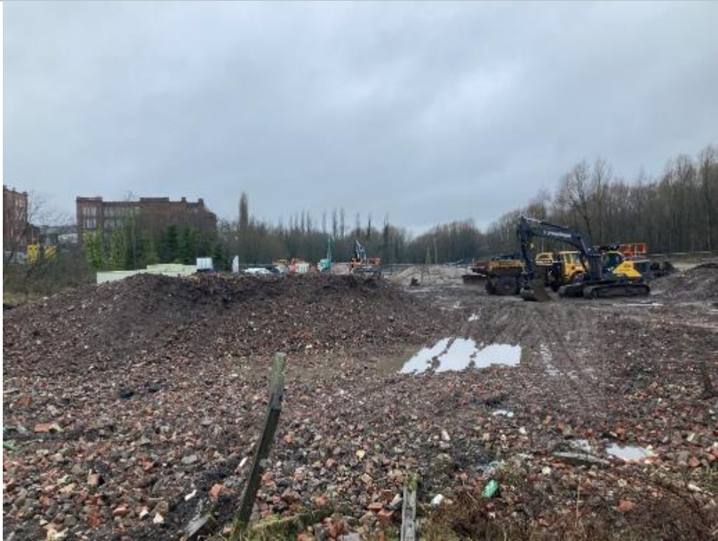
PLATE 29 PROCESSING OF MADE GROUND
