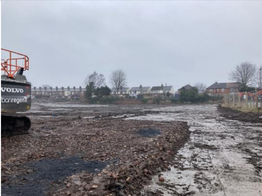
CONSTRUCTION OF TEMPORARY WORKING PLATFORM PHASE 3 (AREA 5)
