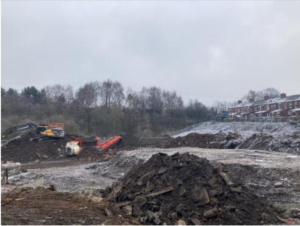
PLATE 31 PROCESSING OF MADE GROUND PHASE 3 (AREA 5)
