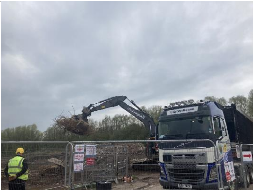
PLATE 48 REMOVAL AND SEGREGATION OF WASTE
