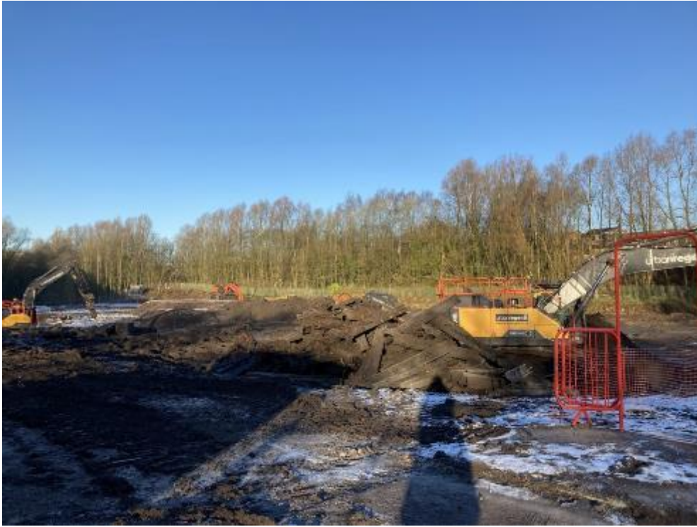
PLATE 33 BREAKING AND PROCESSING OF ABOVE AND BELOW GROUND STRUCTURES PHASE 1 (AREA 1)
