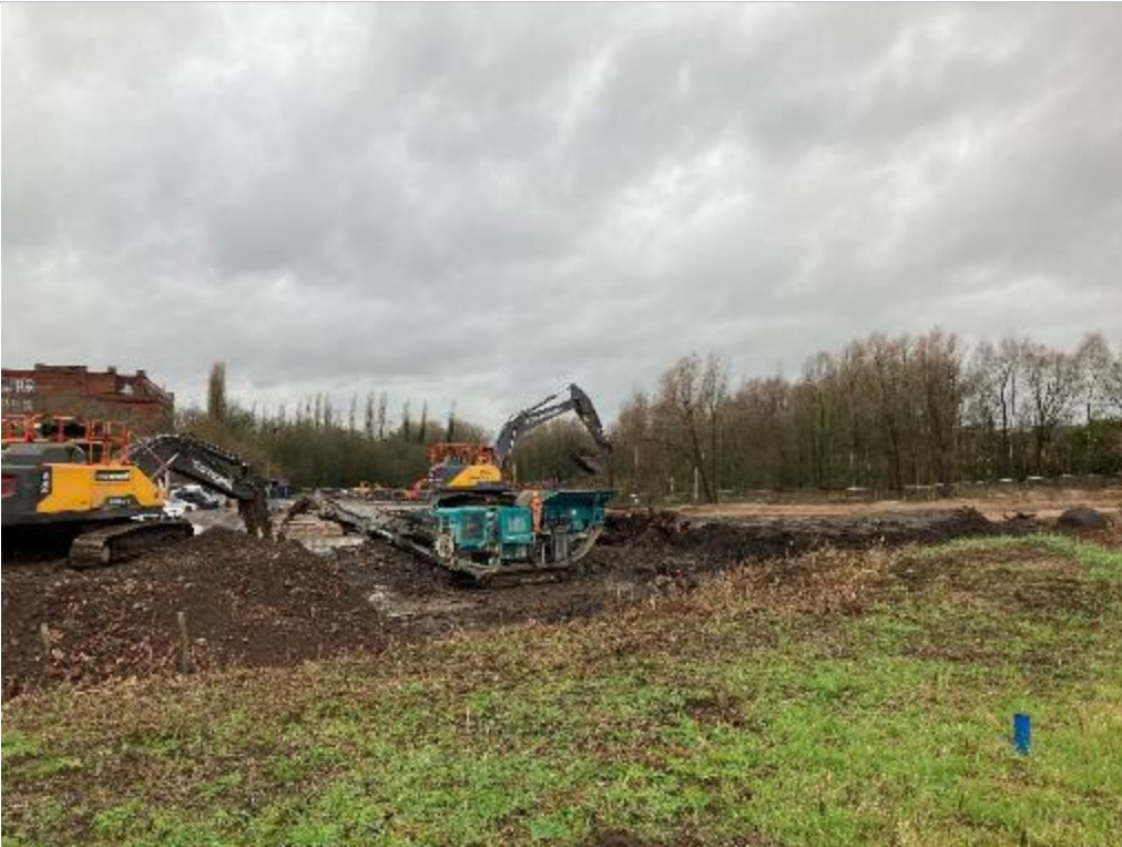
PLATE 34 PROCESSING OF MADE GROUND (AREA 2A)
