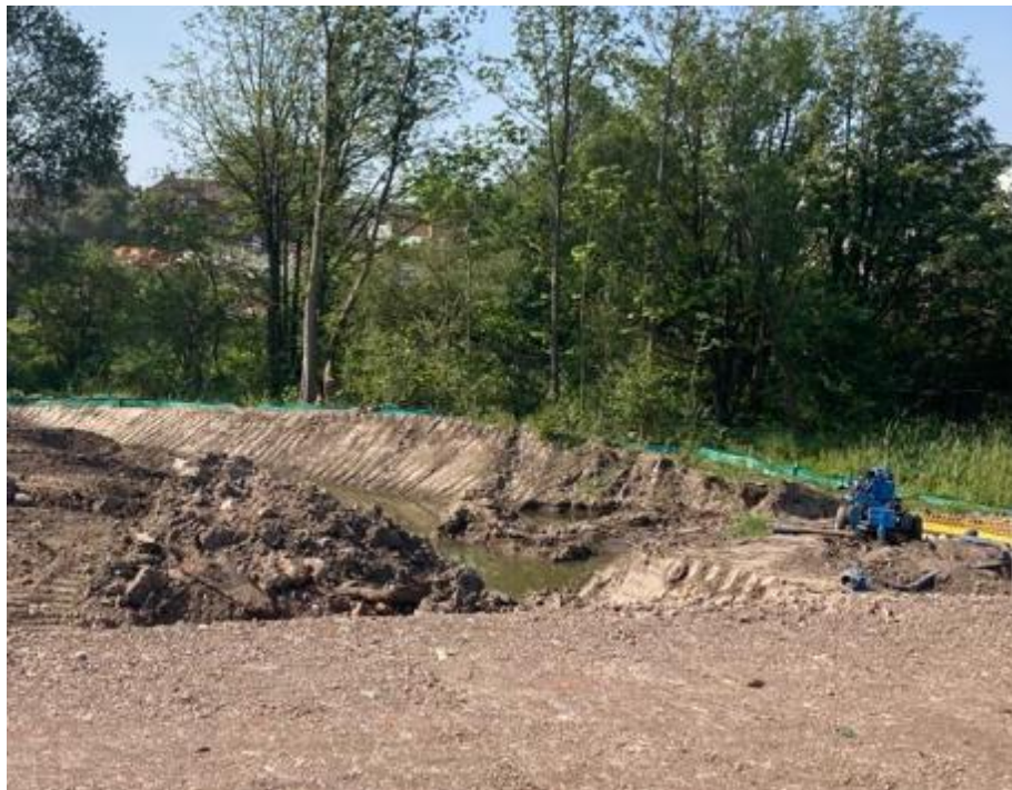
PLATE 6 SILT BUSTER AND FENCING ON SITE DURING EXCAVATION AND DEWATERING
