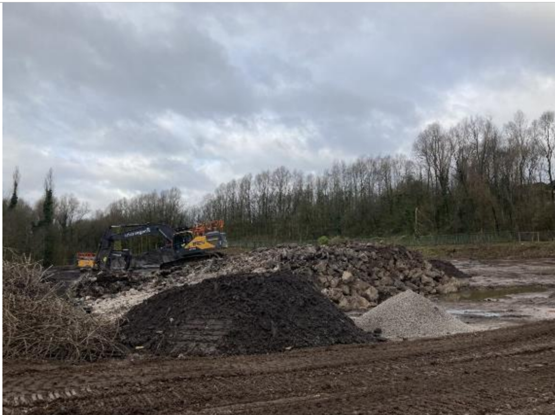
PLATE 30 BREAKING AND PROCESSING OF MADE GROUND
