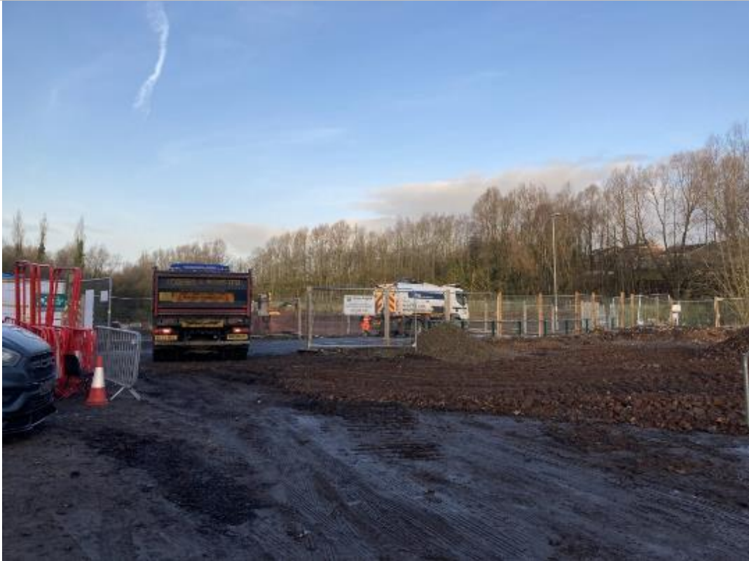
PLATE 59 IMPORTATION OF BULK FILL TO PHASE 2A
