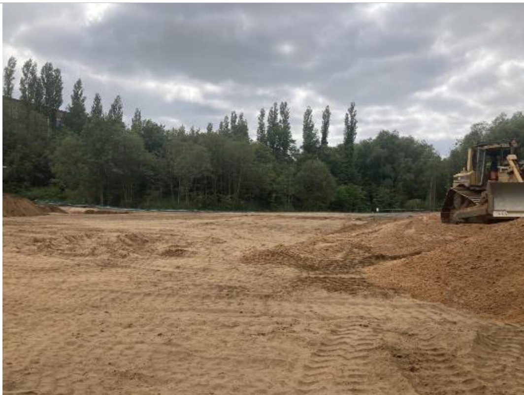
PLATE 54 FILLING OPERATIONS IN PHASE 1 (AREA 1)
