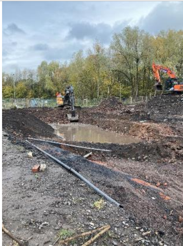
PLATE 35 BREAKING AND PROCESSING OF ABOVE AND BELOW GROUND STRUCTURES PHASE 1 (AREA 2A)
