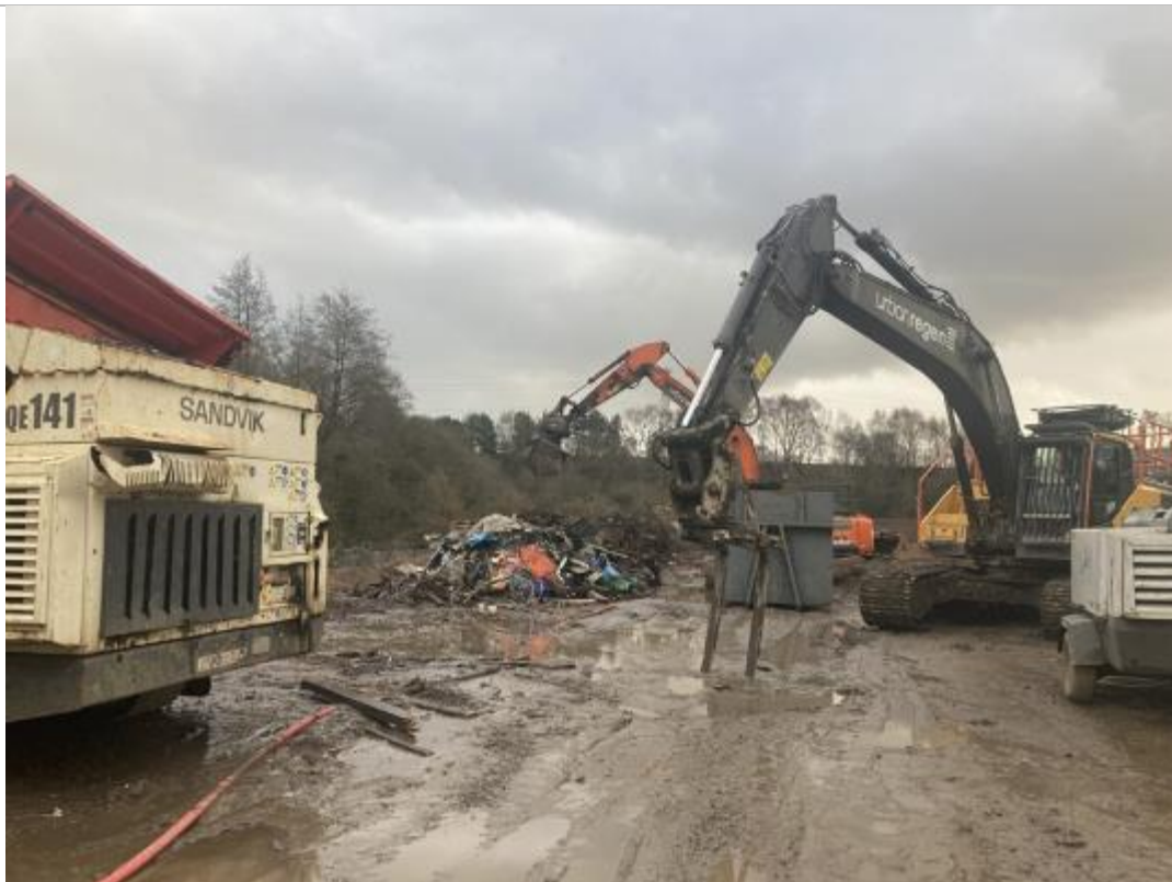
PLATE 46 REMOVAL AND SEGREGATION OF WASTE
