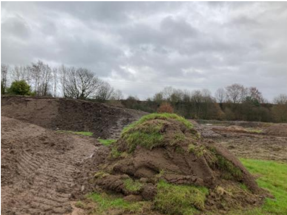
PLATE 15 TOPSOIL AND TURF ARISING FROM AREA 2
