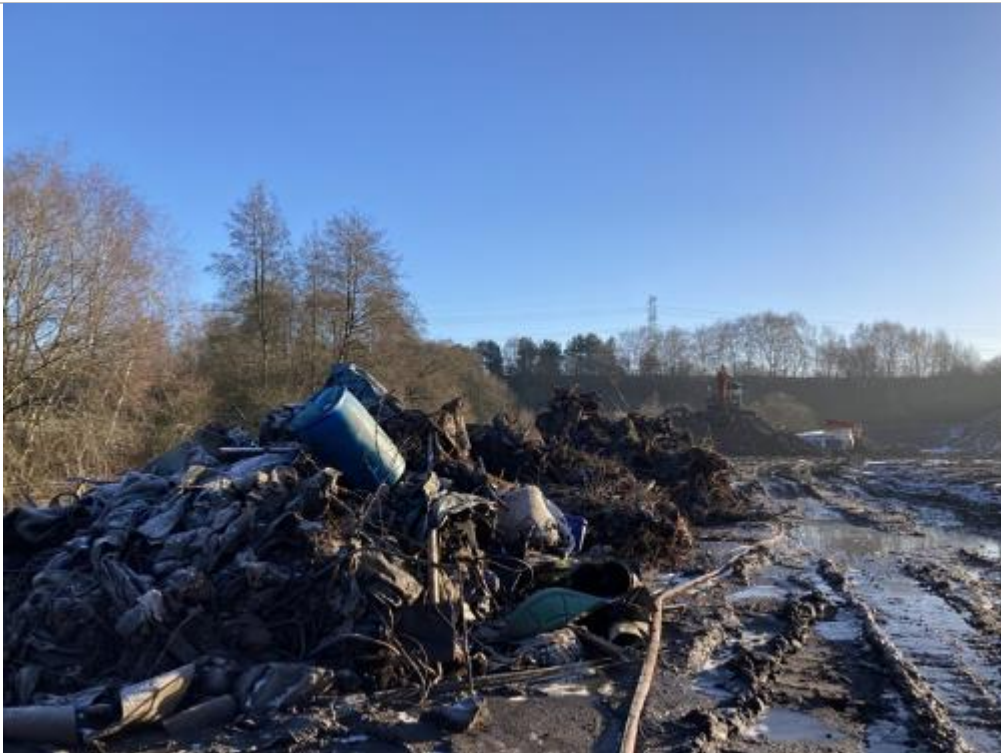
PLATE 44 REMOVAL AND SEGREGATION OF WASTE
