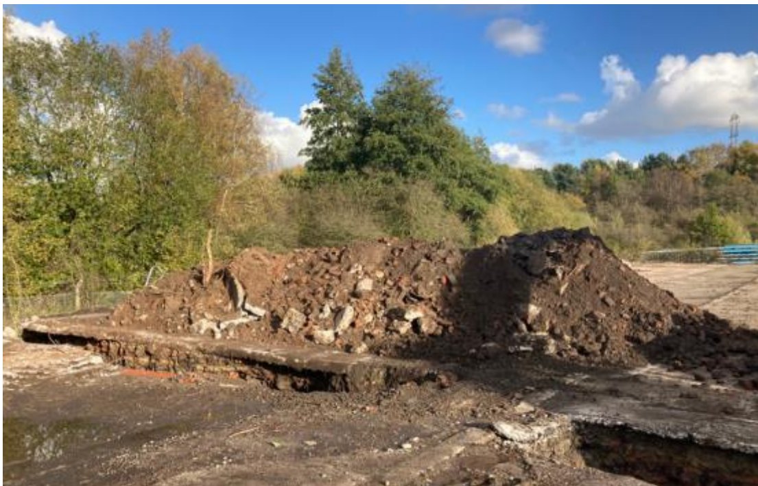
PLATE 12 START OF SLAB REMOVAL IN PHASE 3
