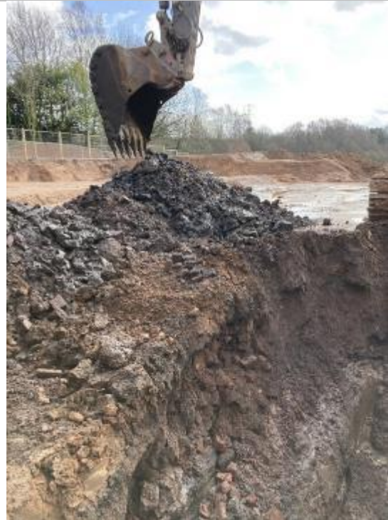
PLATE 41 DELINEATION, EXCAVATION AND TREATMENT OF INFILLED HISTORICAL PONDS AND STREAMS
