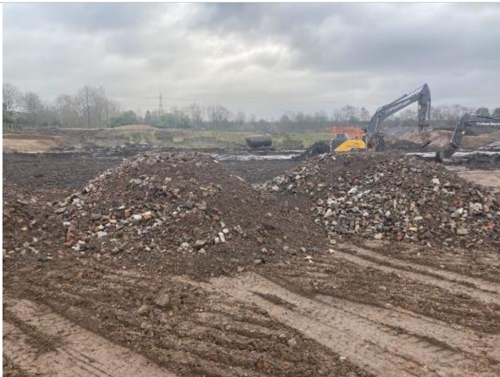
PLATE 28 PROCESSED MADE GROUND FOR RE-USE
