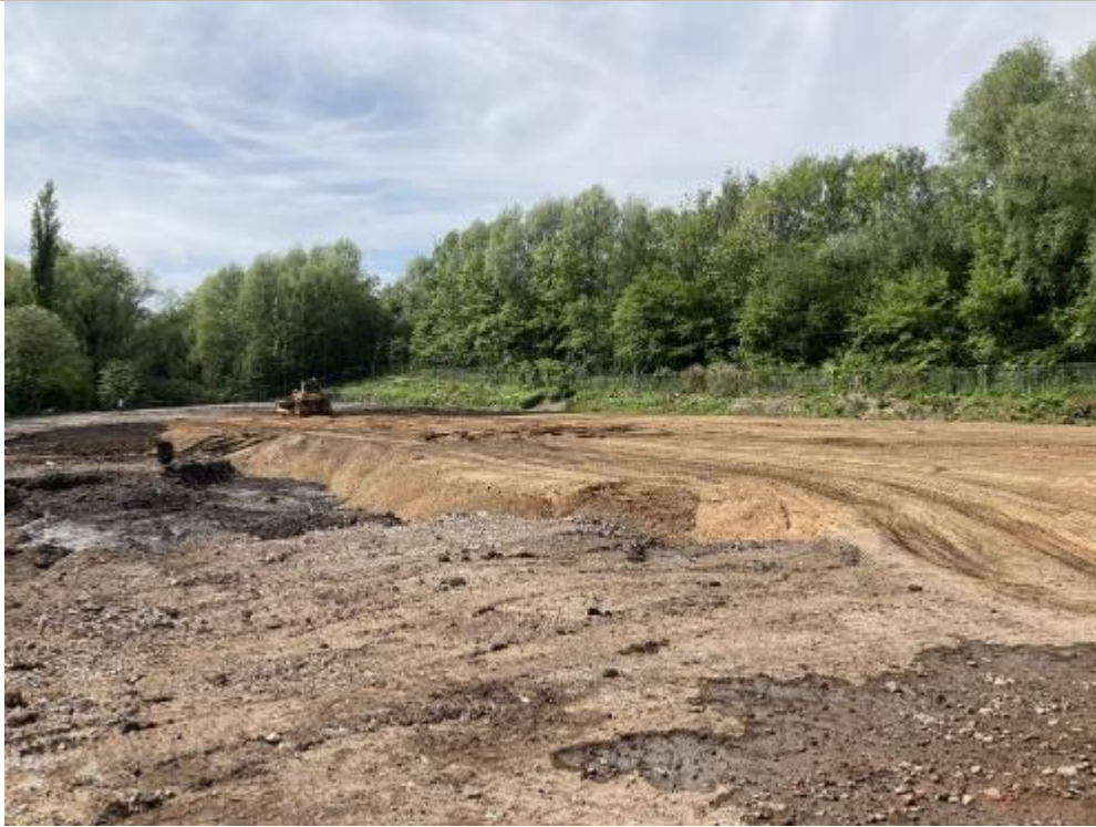
PLATE 55 FILLING OPERATIONS IN PHASE 1 (AREA 1)
