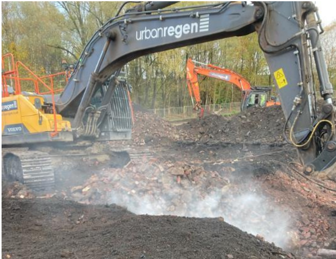
PLATE 11 REMOVAL OF SLAB AND SHALLOW OBSTRUCTIONS WITHIN PHASE 1
