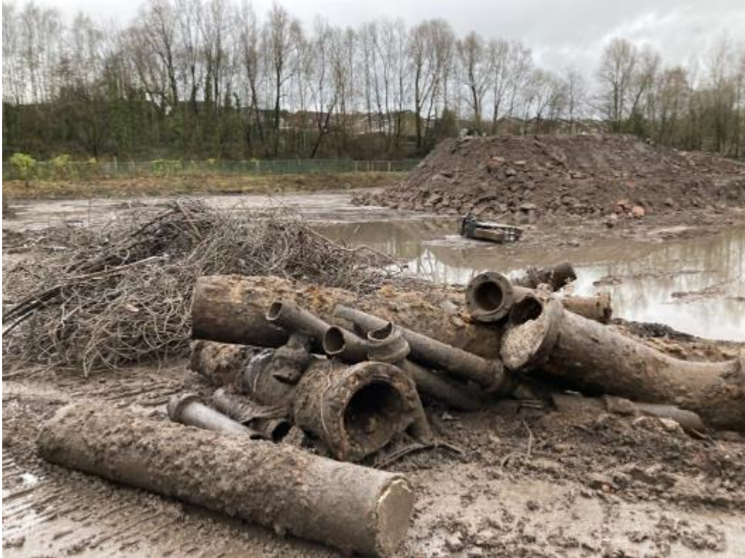
PLATE 45 REMOVAL AND SEGREGATION OF WASTE
