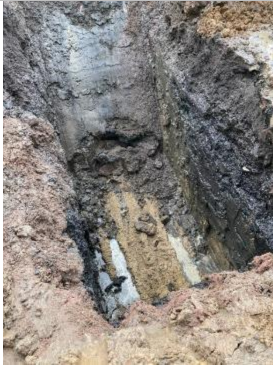
PLATE 41 DELINEATION, EXCAVATION AND TREATMENT OF INFILLED HISTORICAL PONDS AND STREAMS
