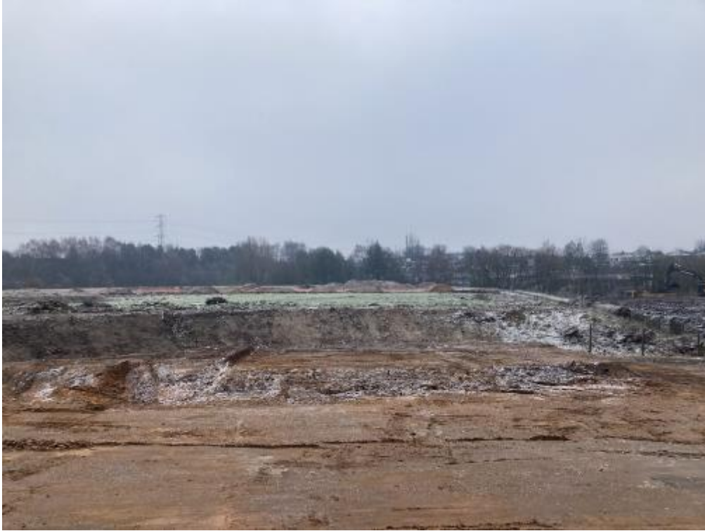
SUPPLEMENTARY TRIAL PITTING PHASE 3 (AREA 5)
