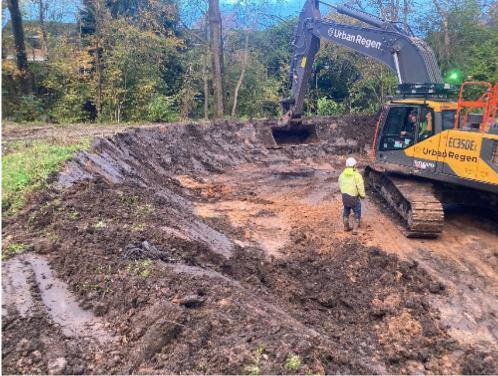
PLATE 43 DELINEATION, EXCAVATION AND TREATMENT OF INFILLED HISTORICAL PONDS AND STREAMS
