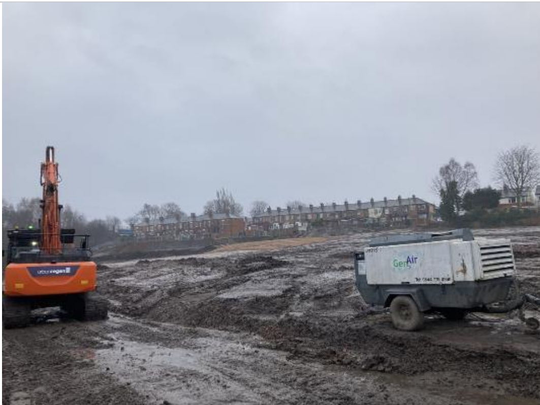
PLATE 56 CUT AND FILL WORKS (AREA 5)
