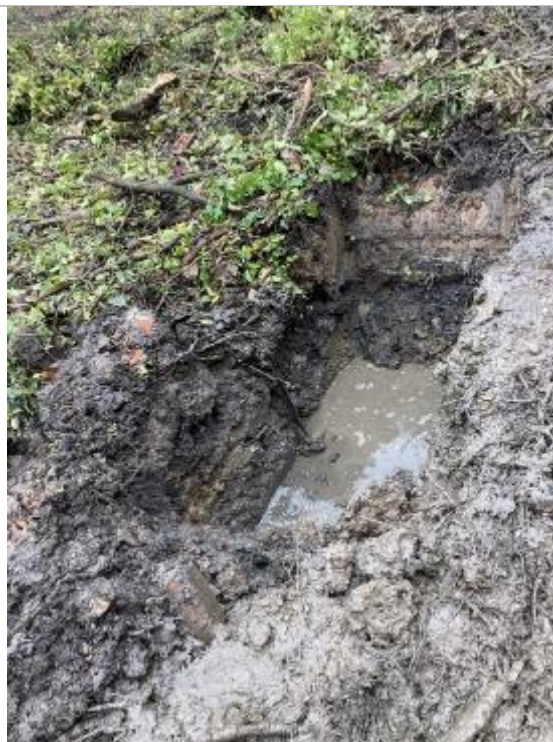
PLATE 38 SUPPLEMENTARY TRIAL PITTING OF IMPACTED SOILS
