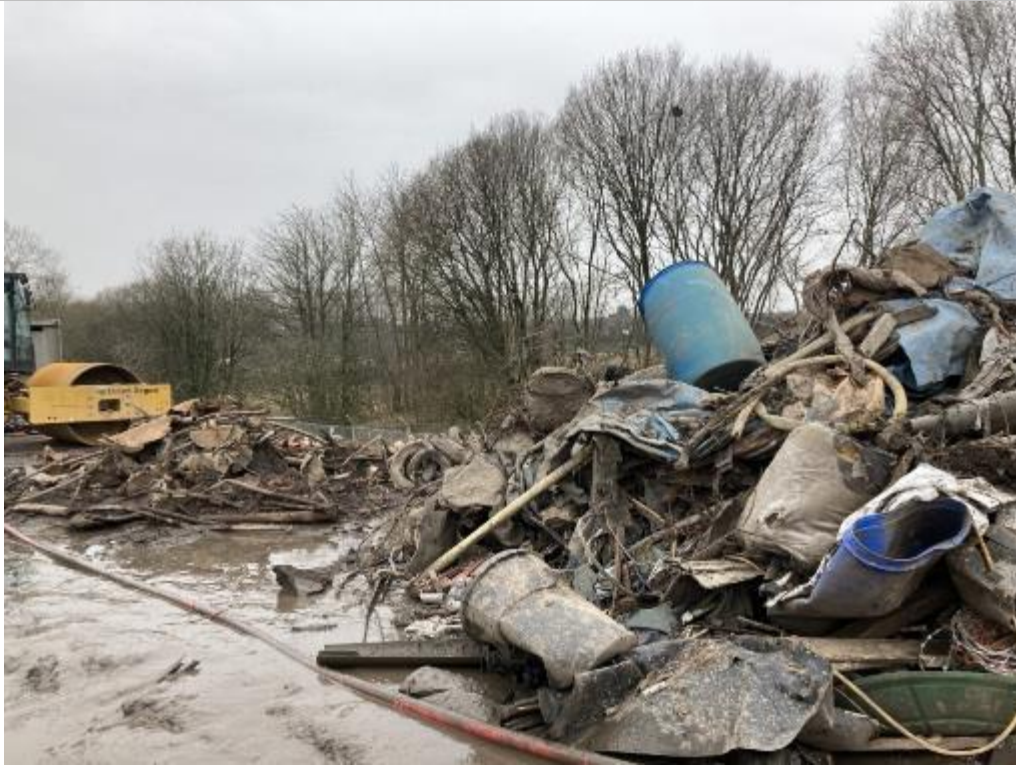
PLATE 47 REMOVAL AND SEGREGATION OF WASTE
