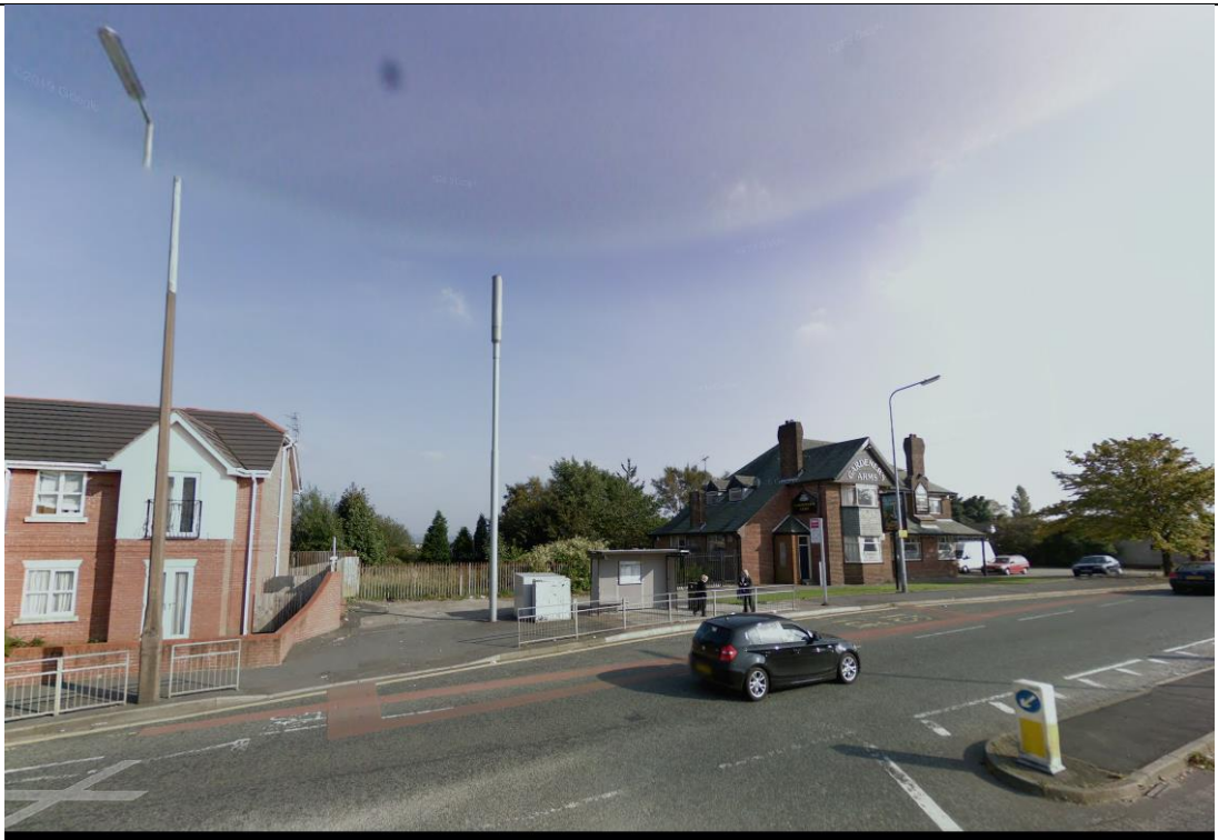
Previous 12.5m monopole at Hollin Lane.
