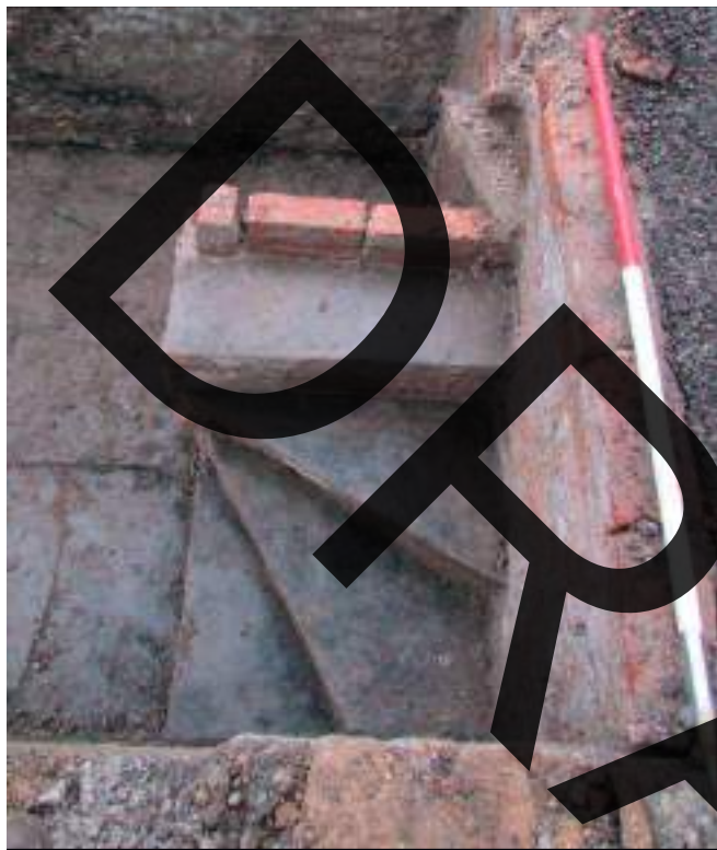
Close-up of cellar steps constructed out of flag stones and brick fireplace
