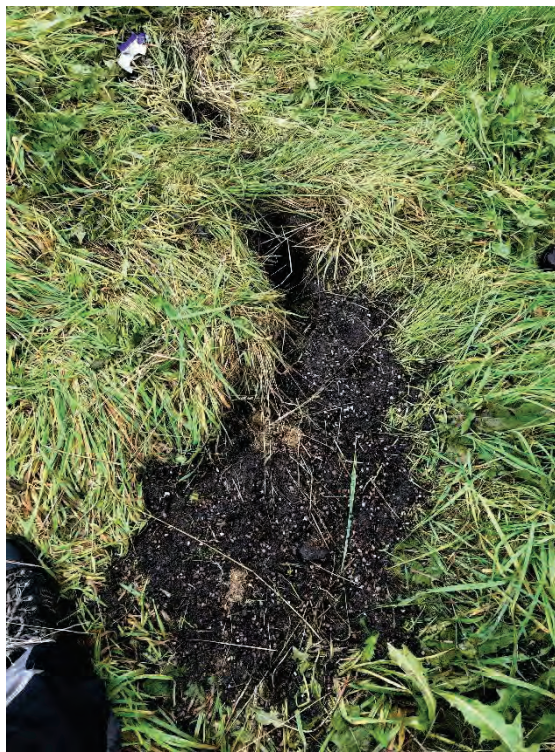
Photo 10: Evidence of infilled ground (2/2)
