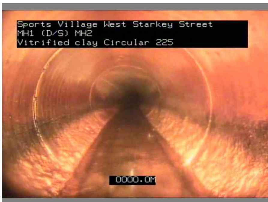
_da90d75e-b133-4cf3-b8f6-96bef0b27ae6.jpg, 00:06:07, 68.40 m Finish survey
