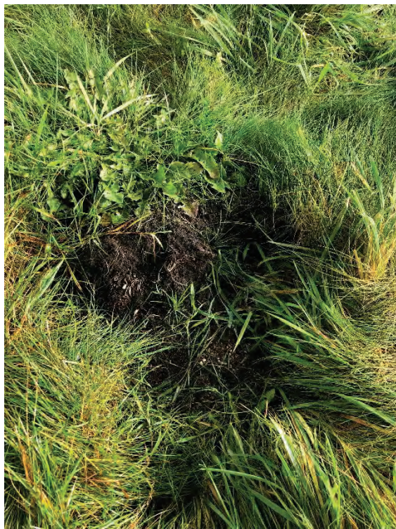
Photo 9: Evidence of infilled ground (1/2)
