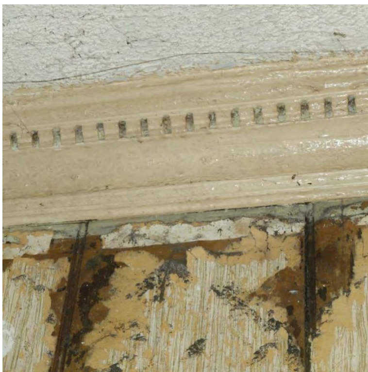
Photo. Timber partition with timber cornice
