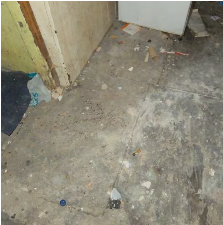
Photo. Suspended York stone floor to ground level Room F.04
