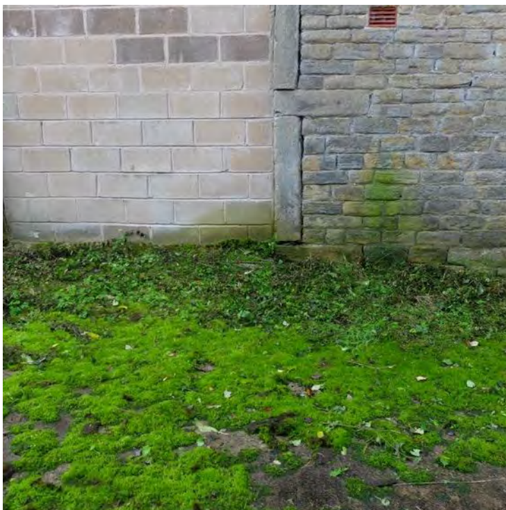
Photo. Repacking of threshing door reveals
