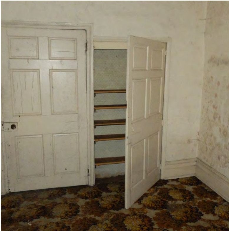
Photo. Door with G.06 and cupboard
