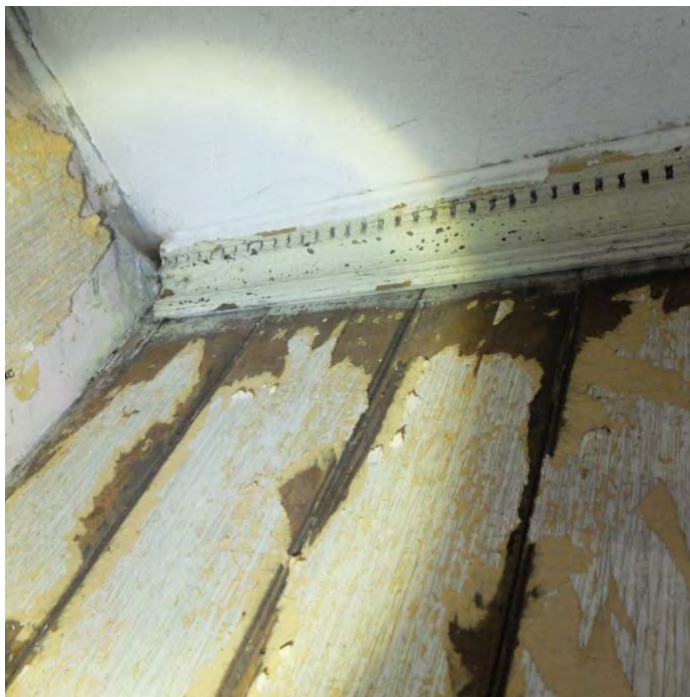
Photo. Timber partition with cornice
