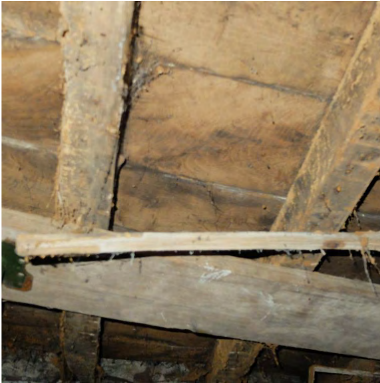
Photo. Ceiling in basement
