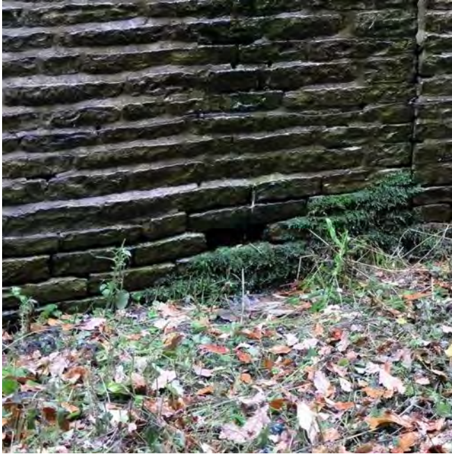
Photo. Air vent in front elevation
