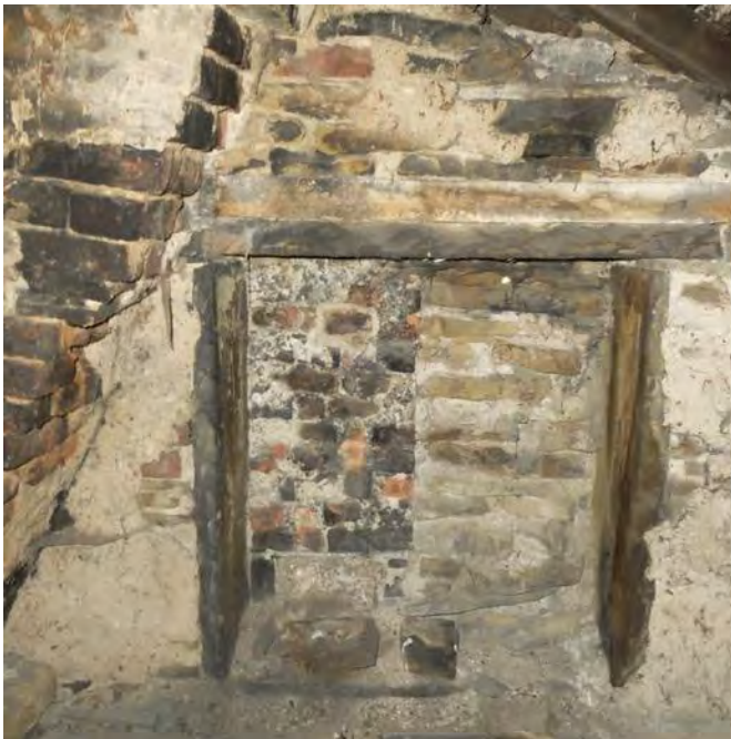
Photo. Old window infilled with masonry.
