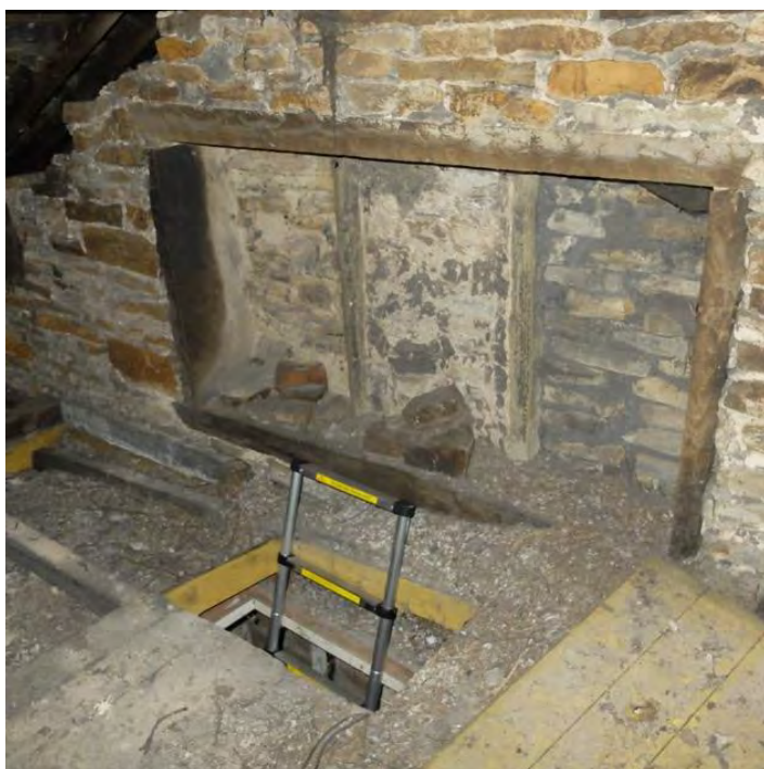
Photo. Infilled window to east gable.
