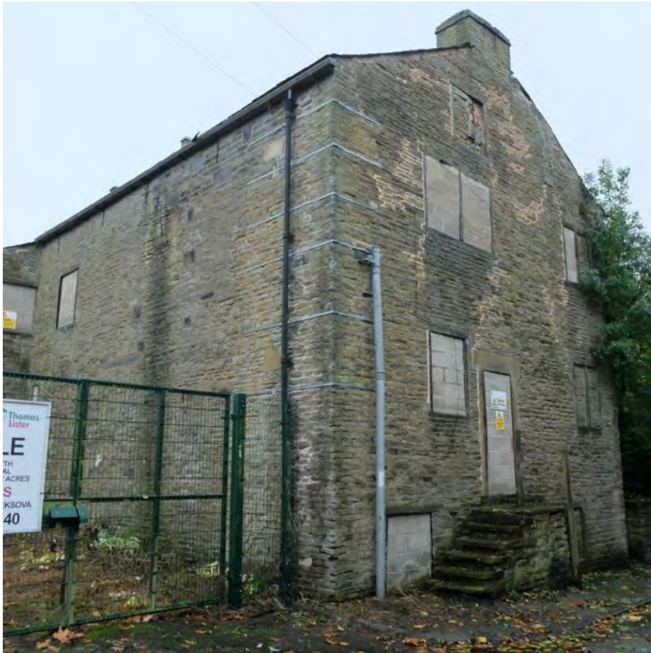
Photo. Full view of gable which overlooks road
