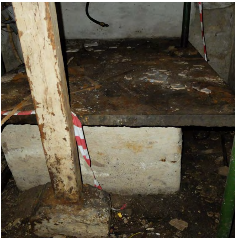
Photo. Stone table to basement
