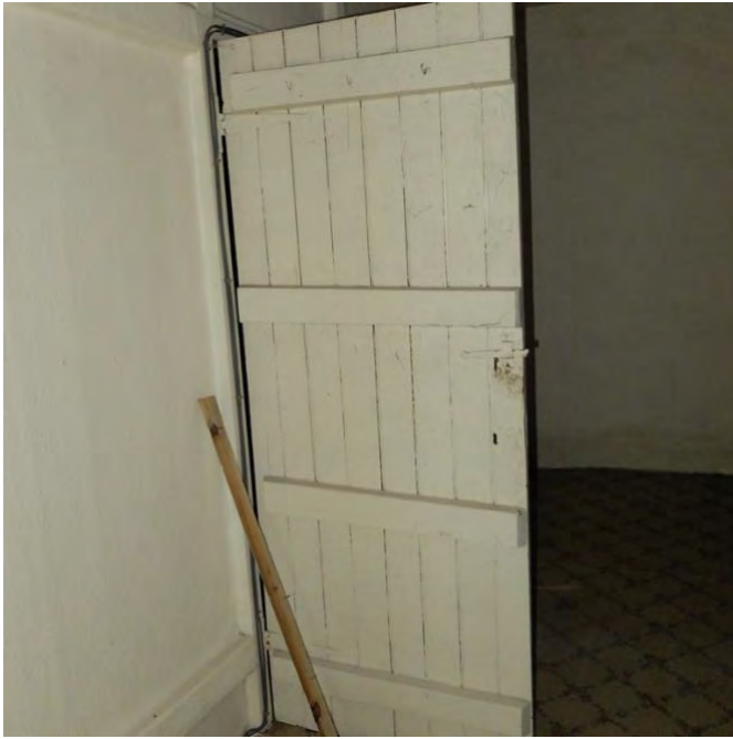
Photo. Timber door to bedroom
