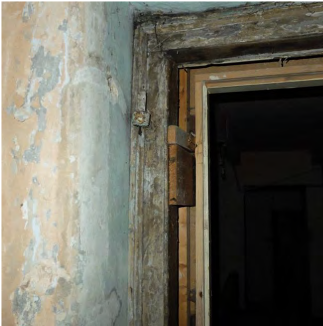
Photo. Old door frame to landing
