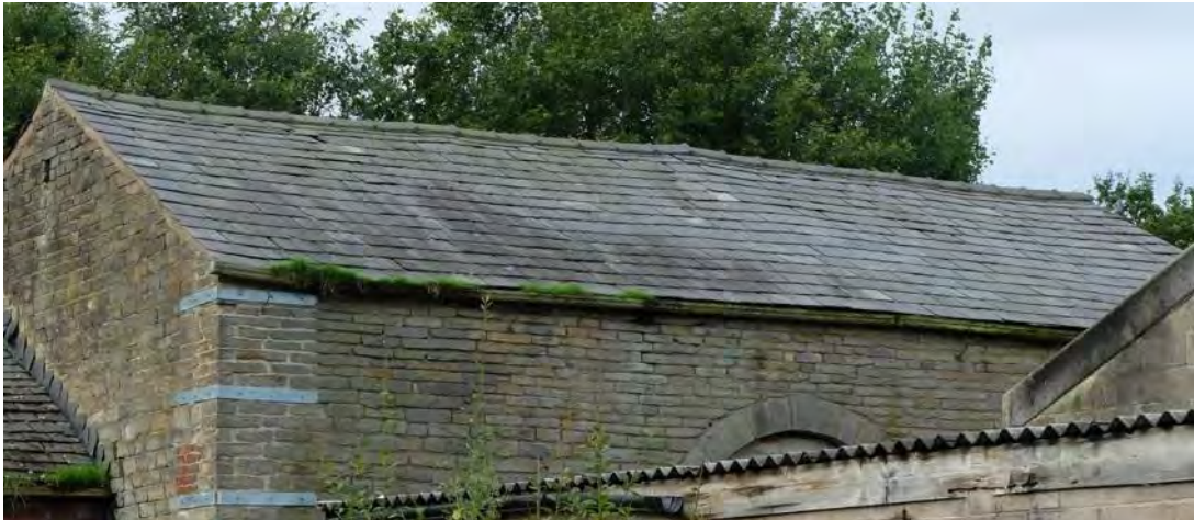
Photo. diminishing coursed slate roof over barn
