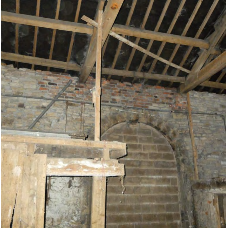
Photo. Rebuilding inner leaf in. brickwork
