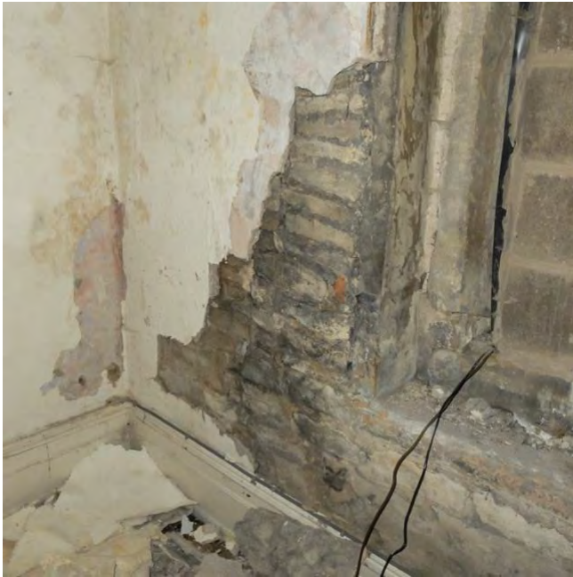
Photo. Added plaster from elevation Room G.03
