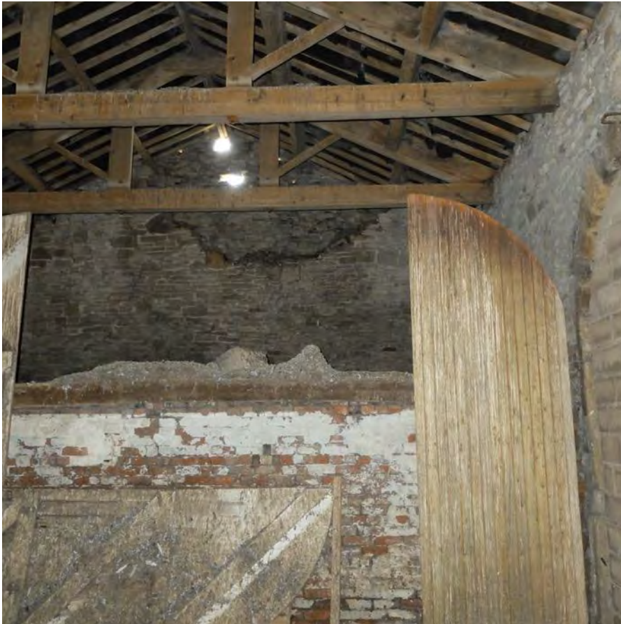
Photo. Threshing barn doors
