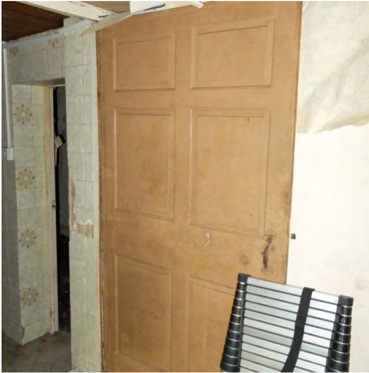
Photo. Original door to hall
