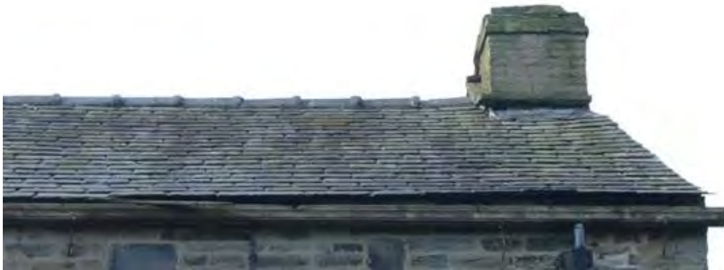
Photo. Diminishing coursed slate roof to farmhouse
