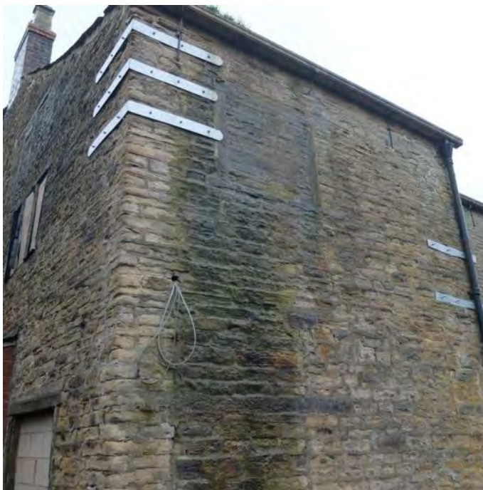
Photo. Corner straps to high level.
