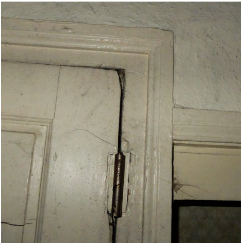
Photo. Moulded architrave to door
