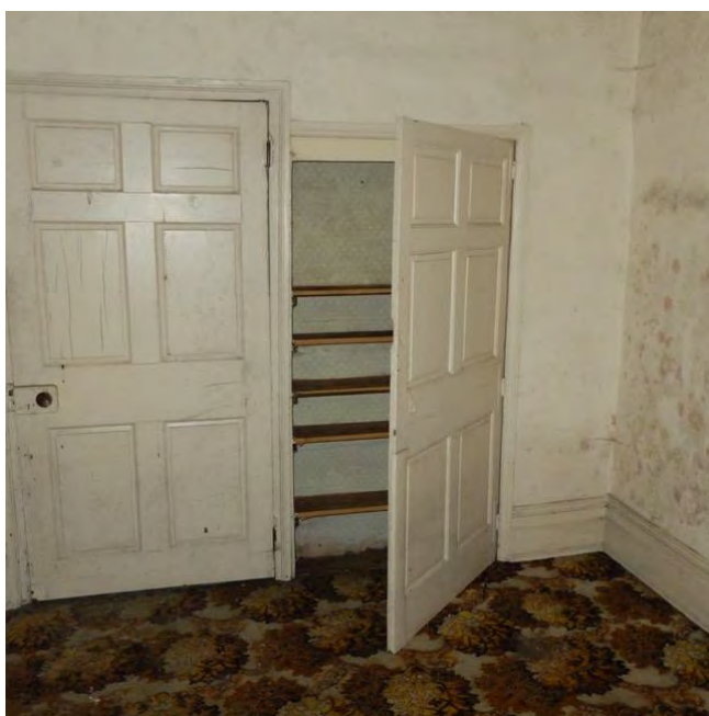
Photo. Original doors to farmhouse Room G.03
