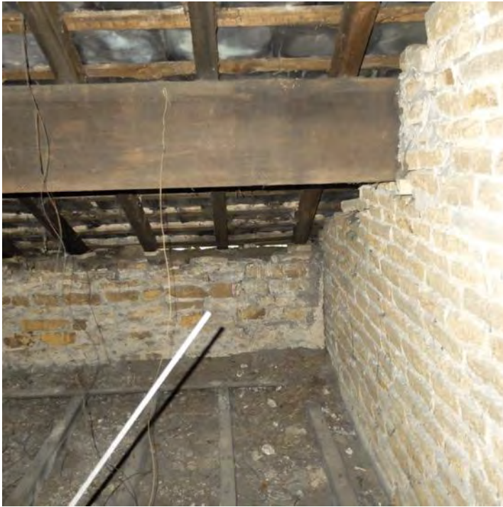
Photo. Rafters sit on wall head no fixing.
