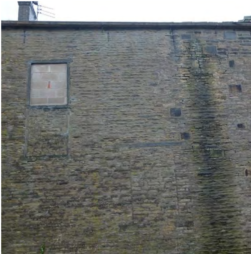
Photo. Infilled windows to rear elevation.
