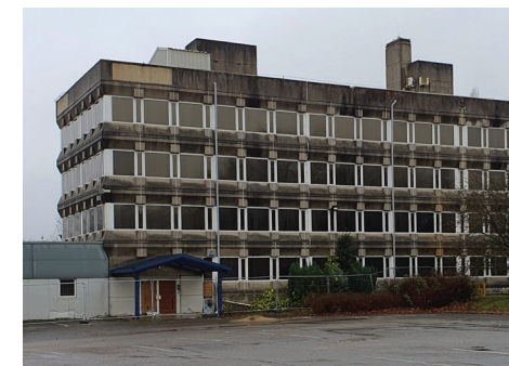
8. Parkfield House - The Modernist/Brutalist building offers a contrast in architectural style from the other buildings within the CA.
