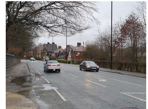
5. Manchester Old Road - Fast moving and wide vehicular road resulting in car dominance over pedestrians, negatively impacting adjacent heritage assets. The stone retaining wall bounding Parkfield House, whilst being visually attractive, exaggerates the feeling of being 'hemmed in' and not wanting to stop, due to it's height.
