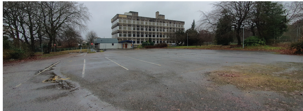
4. Large expanses of hard standing - The tarmac car park serving Parkfield House creates dead space within the CA and detracts from the adjacent heritage assets. This space, with its historic past and elevated position, could be better utilised as a quality piece of public realm whilst also improving pedestrian experiences and connections to Limefield Leisure Park.
