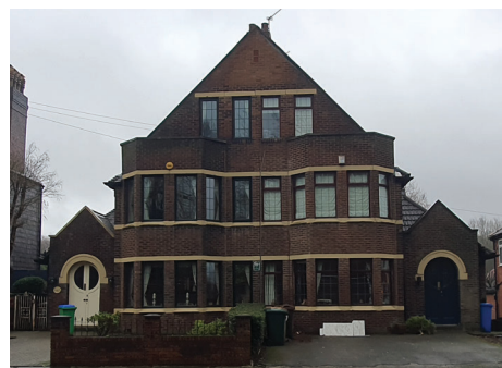
4. 161-163 Manchester Old Road - Semi detached houses which stands out as a landmark due its material composition and form, also aligns with the building line along Manchester Old Road.
