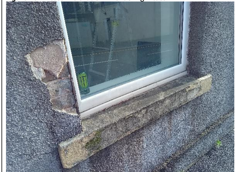
Figure 11. Western elevation – windowsills.
