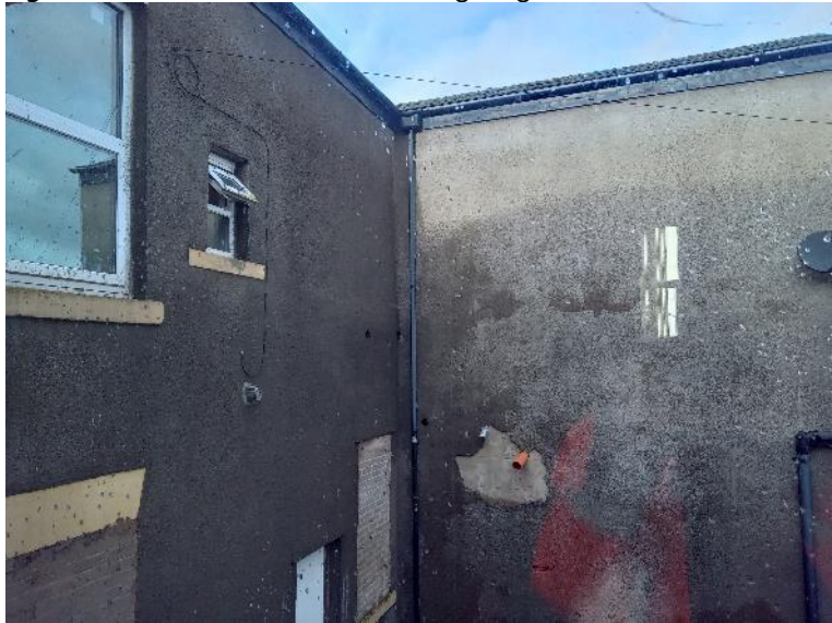
Figure 21. Eastern elevation - 'U' shaped section of B1.
