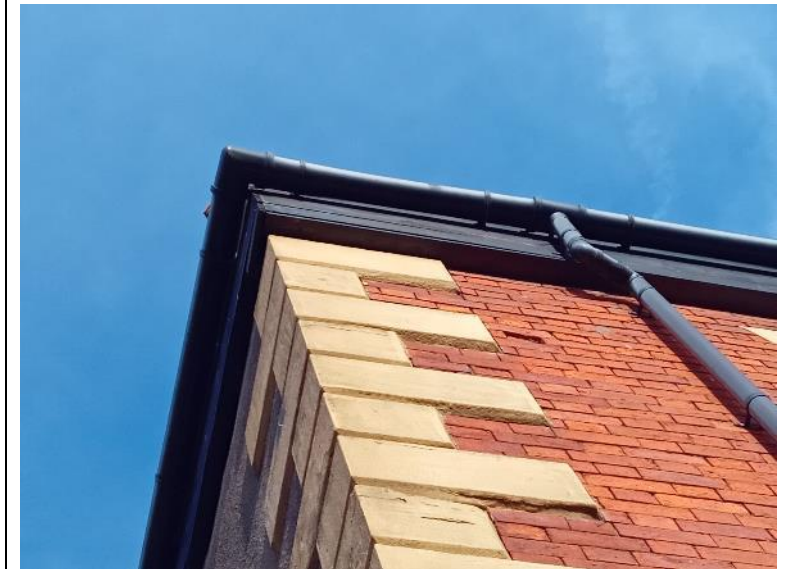
Figure 7. Southern elevation – fascias tightly fitted.
