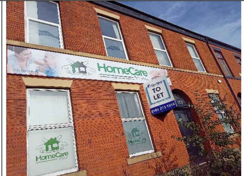
Figure 6. Southern elevation – supporting wall intact.
