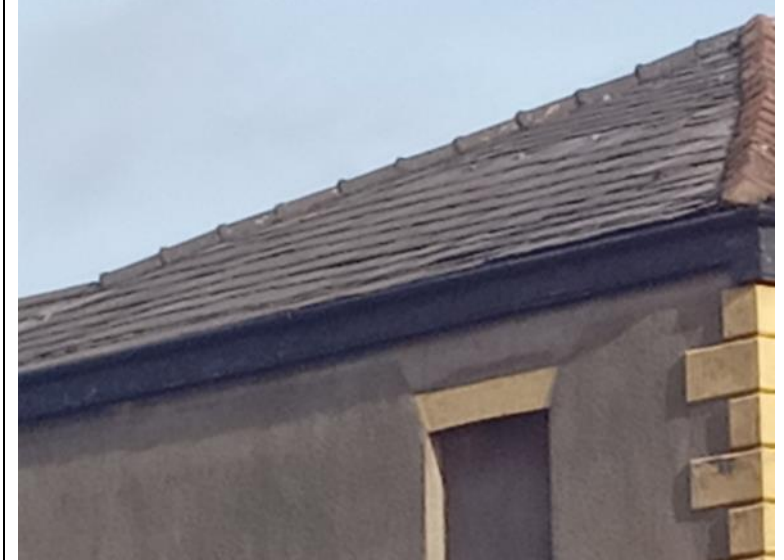
Figure 13. Western elevation – raised tiles.
