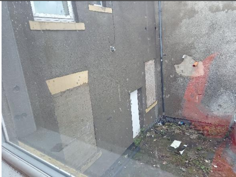
Figure 22. Eastern elevation – ground-level windows filled.
