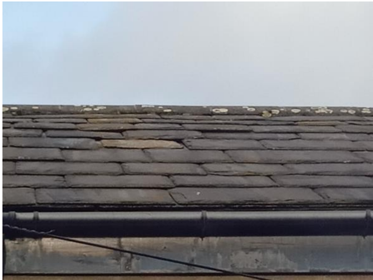
Figure 23. Eastern elevation – raised tiles.
