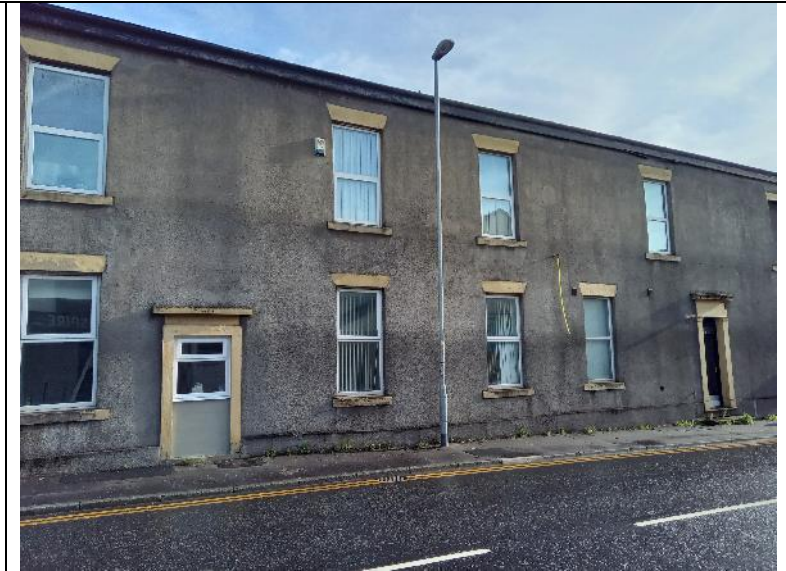
Figure 10. Western elevation – rendering intact.
