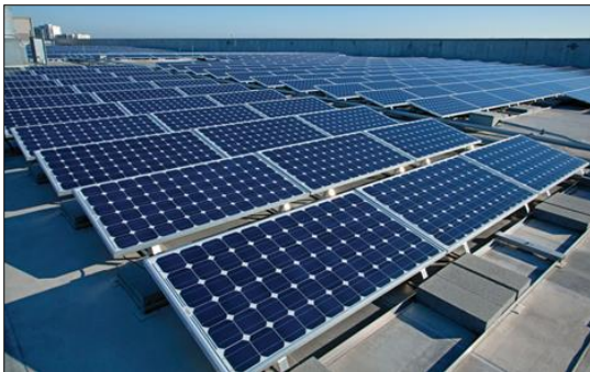
Figure 11. Solar panels installed to flat roof 5
