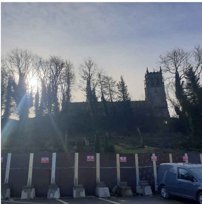
Photograph 1: area of work on arrival at site
