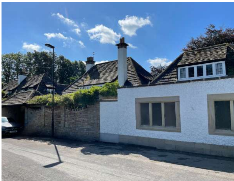
Figure 4.7: No 15 Broadhalgh Avenue
