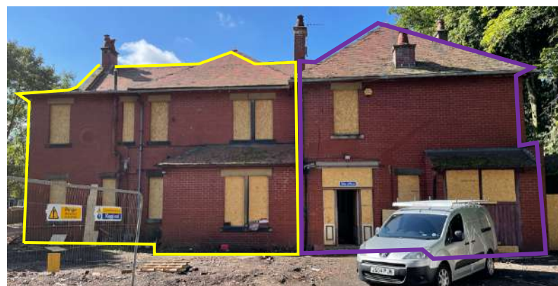
Figure 4.10: Front Elevation to the Red House
