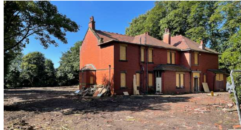
Figure 3.2: Front Elevation to the Red House
