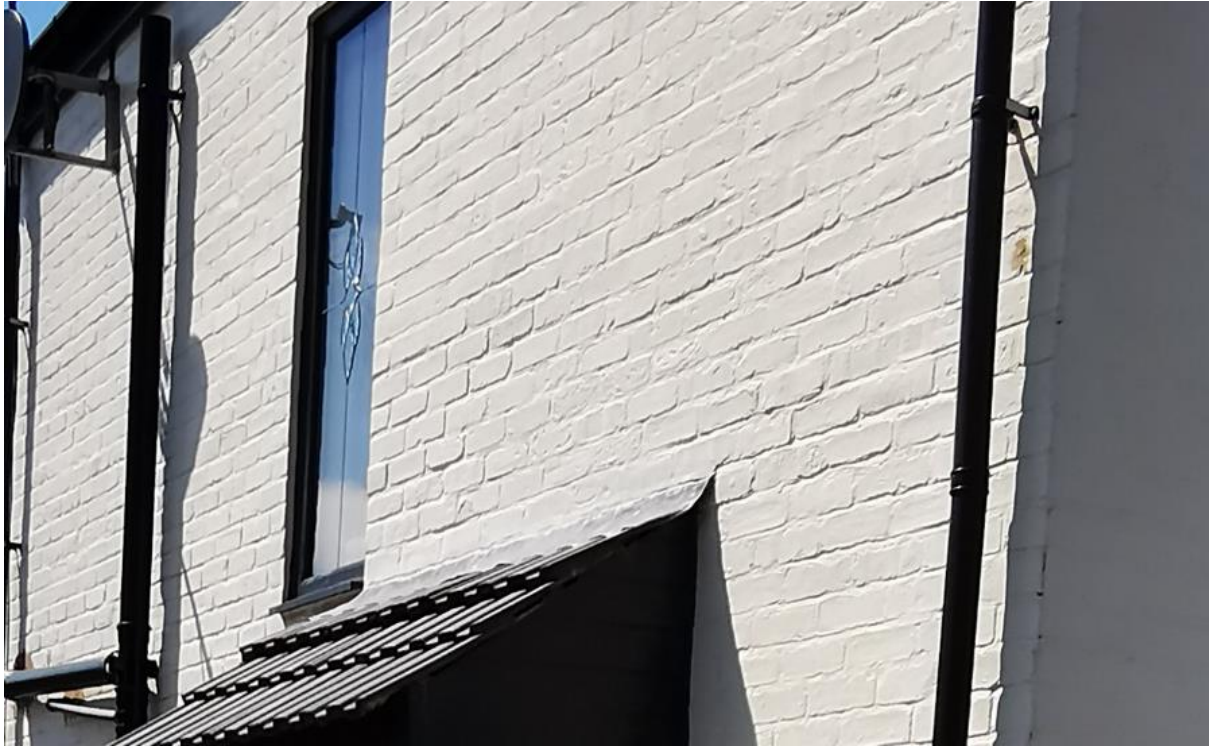
Fig 18. Close up of painted brick work (HAD&Co 2021)
