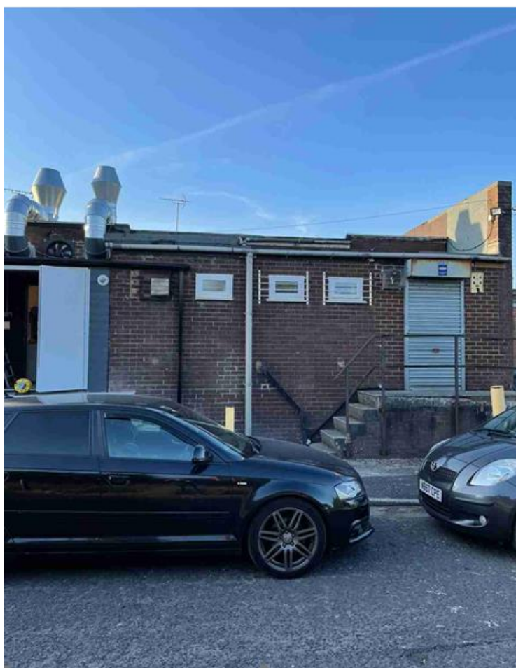
Above image shows the rear of the retail unit, a new flue would be erected
