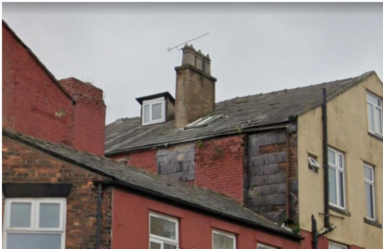
Above image shows dormer and rooflight on adjacent building
