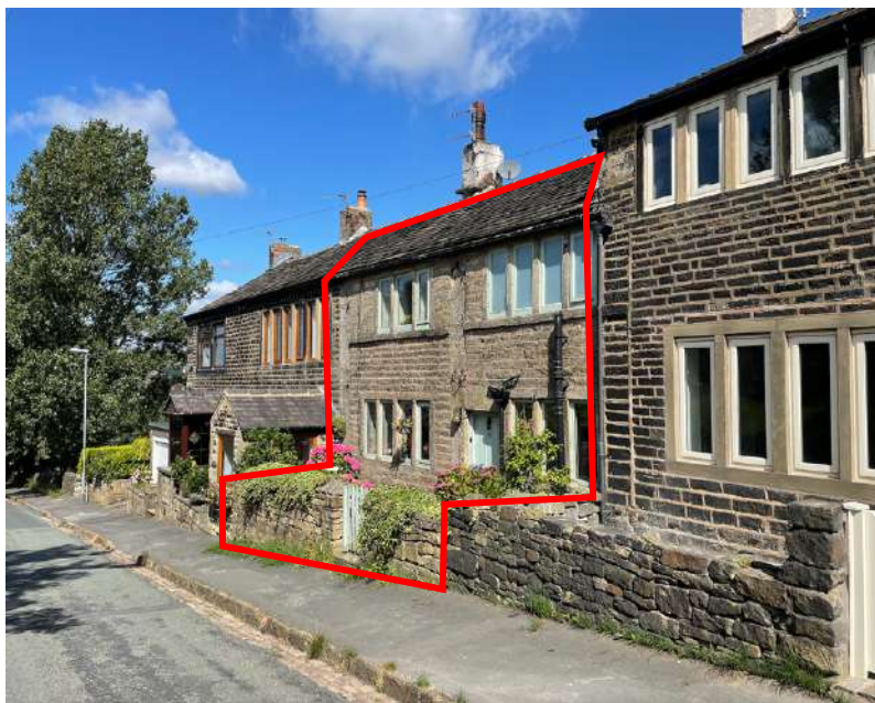
Figure 4.1: No. 5 Blackstone Edge Old Road (August 2022)
