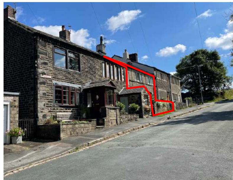
Figure 4.2: No. 5 Blackstone Edge Old Road (August 2022)
