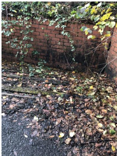
Image 12: Black staining on the wall of the south-western corner.
