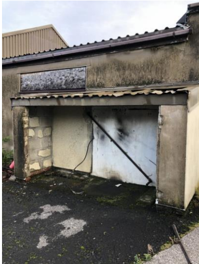
Image 10: Black staining along the western wall of the rear building.
