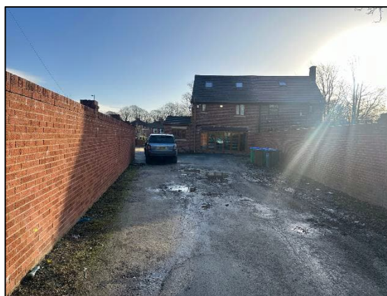
Figure 3.2: Unvegetated garden at entrance to the site to the north
