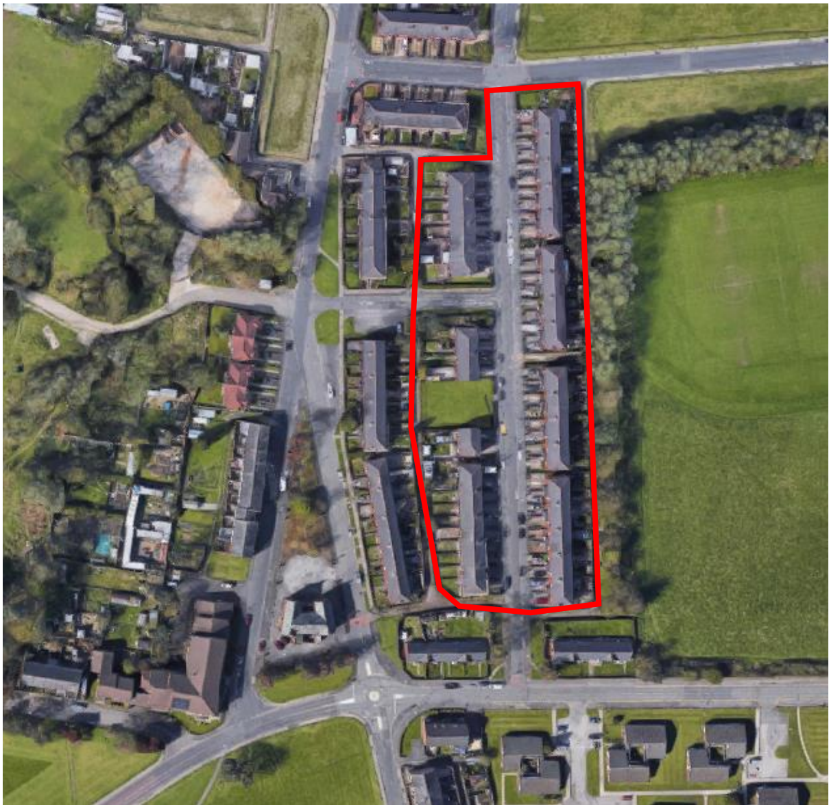
Above – general area of proposed works to north of Heywood town centre
