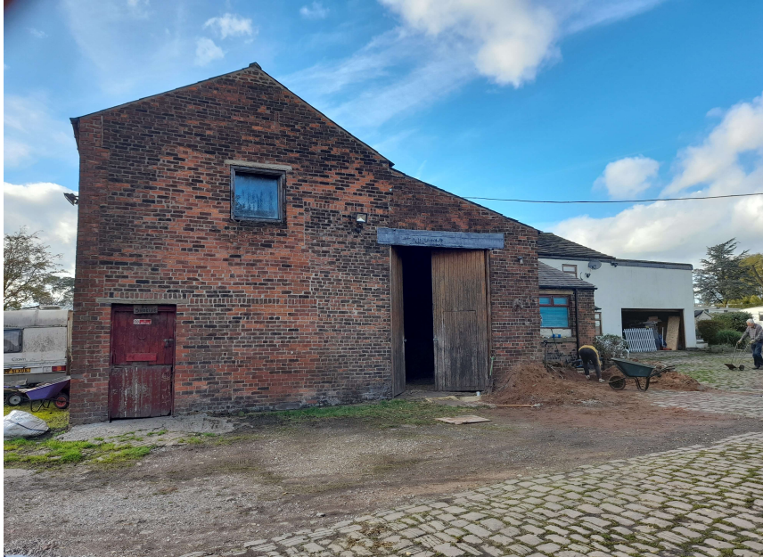
Adjoining barn on east elevation
