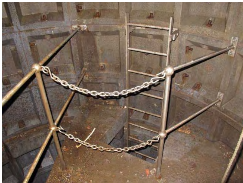
View of Access Ladder to Level 3, Hand Rails and Safety Chains.
