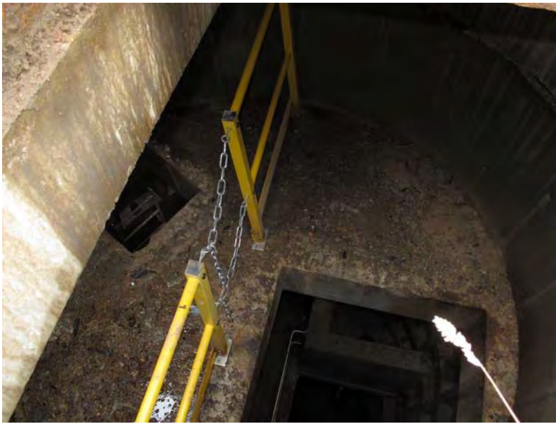
Views from Surface Level to Level 1 and Chamber Base
