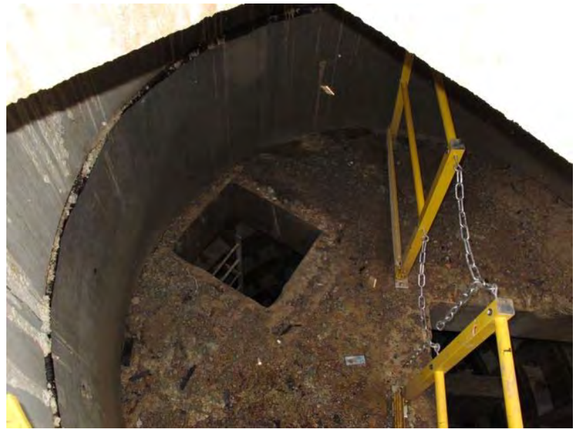
Views From Surface Level to Level 1 Landing
