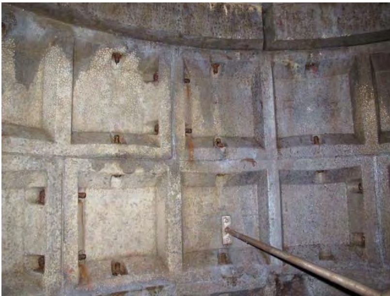
Views of MH Walls at Level 3
