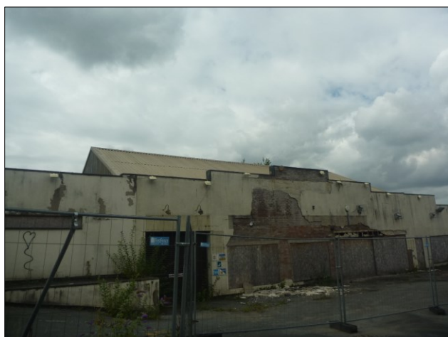
Photo 3: Building 1, north-eastern elevation, southern end
