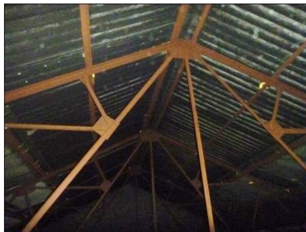
Photo 8: Building 1, void over main showroom
