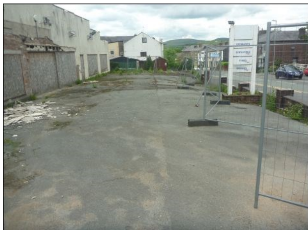
Photo 1: Hard standing with colonising ruderal herbs and north-eastern elevation
