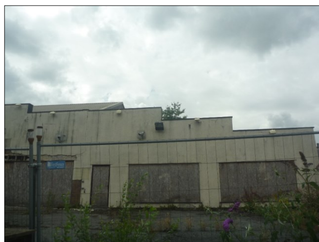
Photo 2: Building 1, north-eastern elevation, northern end
