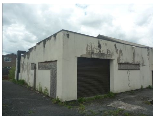
Photo 4: Building 1, eastern corner
