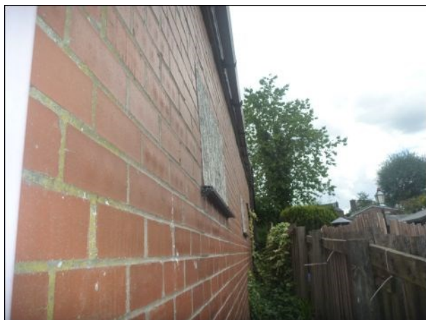
Photo 7: Building 1, north-western elevation
