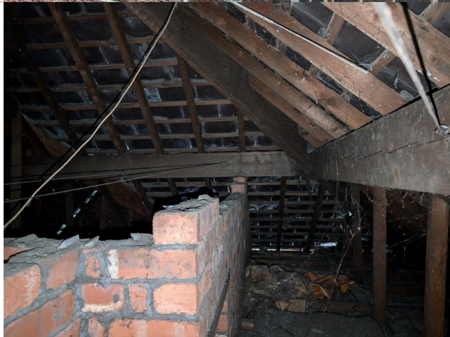
Photos 8a & 8b. Photos of loft and underside of roof.
